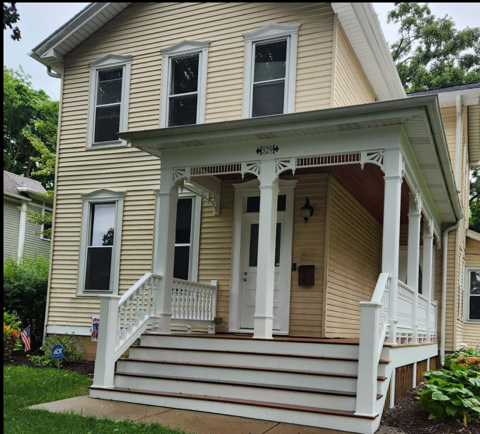
Front Porch after Grant Funded Restoration
