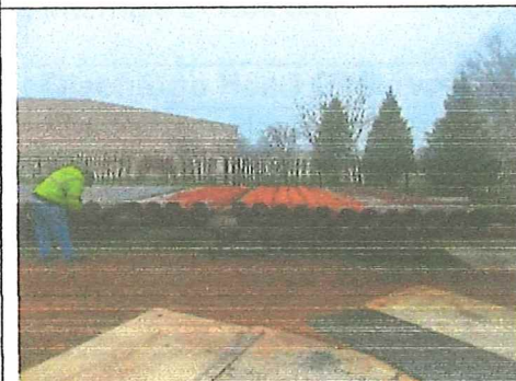
The seventeen lowest pipe joint, on right, were submerged under static water level. Build up is too heavy to determine pipe integrity prior to sand blast.
