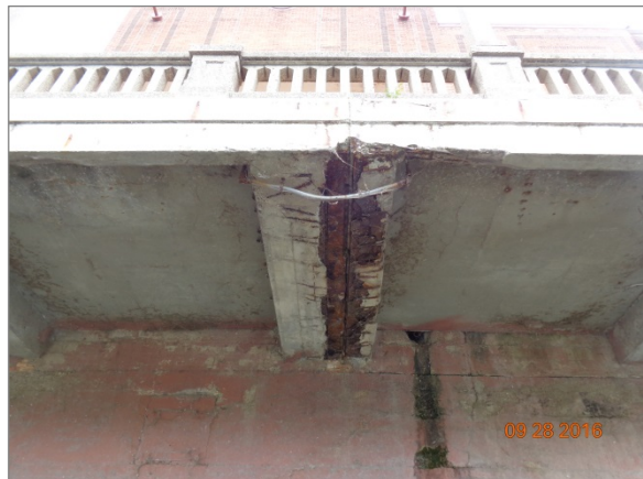
Underside of Expansion Joint
