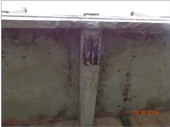
Exposed Beams North of Joint
