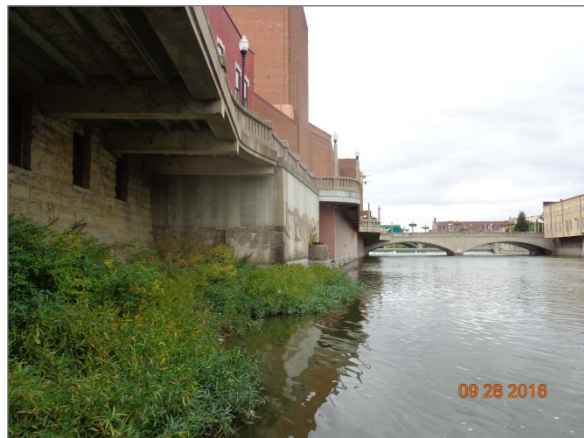
Overall Underside View
