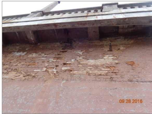
Cantilever Underside at Paramount Auditorium
