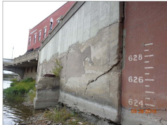
Slab on Grade River Wall
