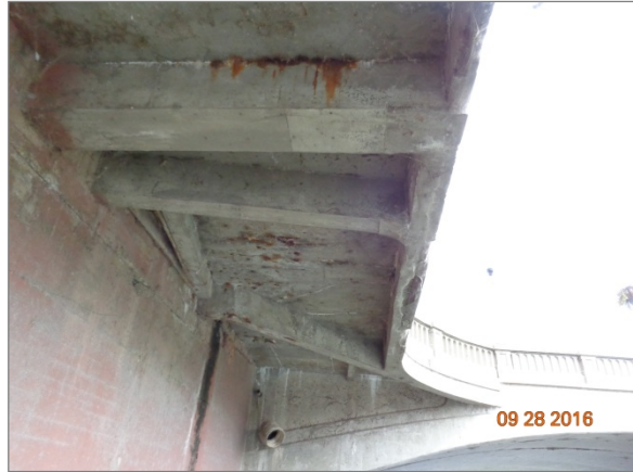
Underside near Galena Bridge
