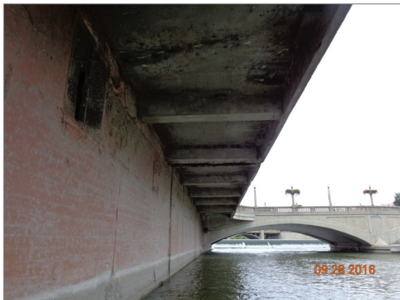
Cantilever Underside at Paramount Lobby
