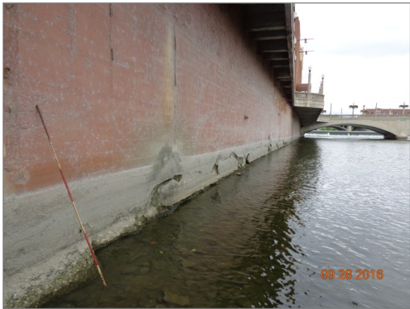
Paramount River Wall
