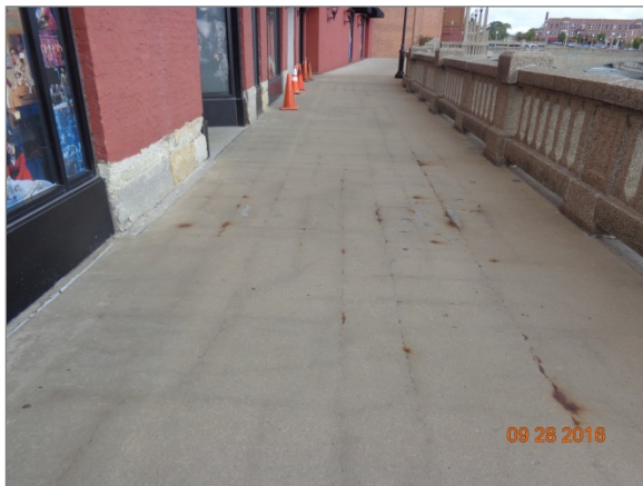
Downer Cantilever Topside
