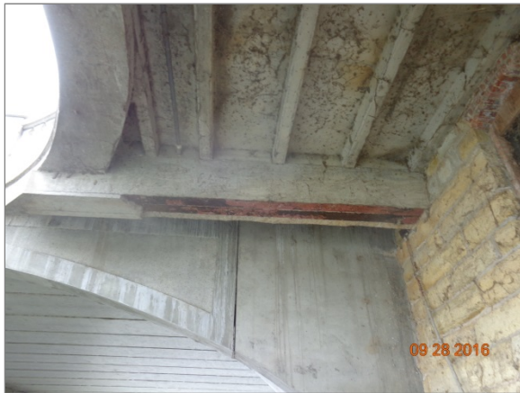
Downer Underside at Bridge
