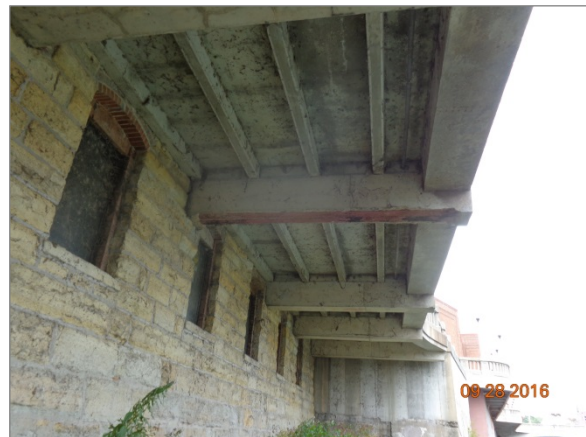
Downer Cantilever Underside
