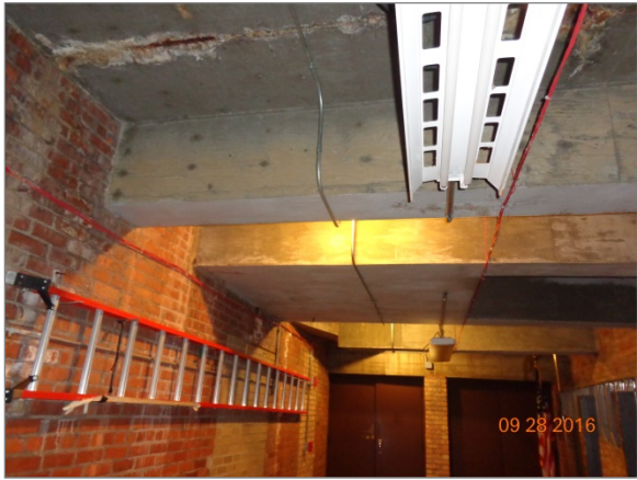
Back Span Underside at Paramount Auditorium
