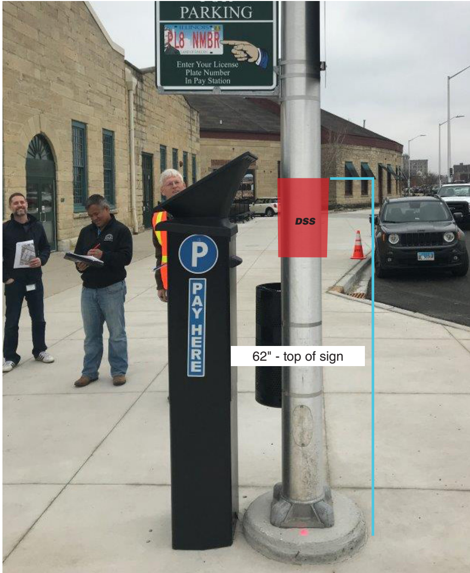
New sign panel mounts to existing street light post.
