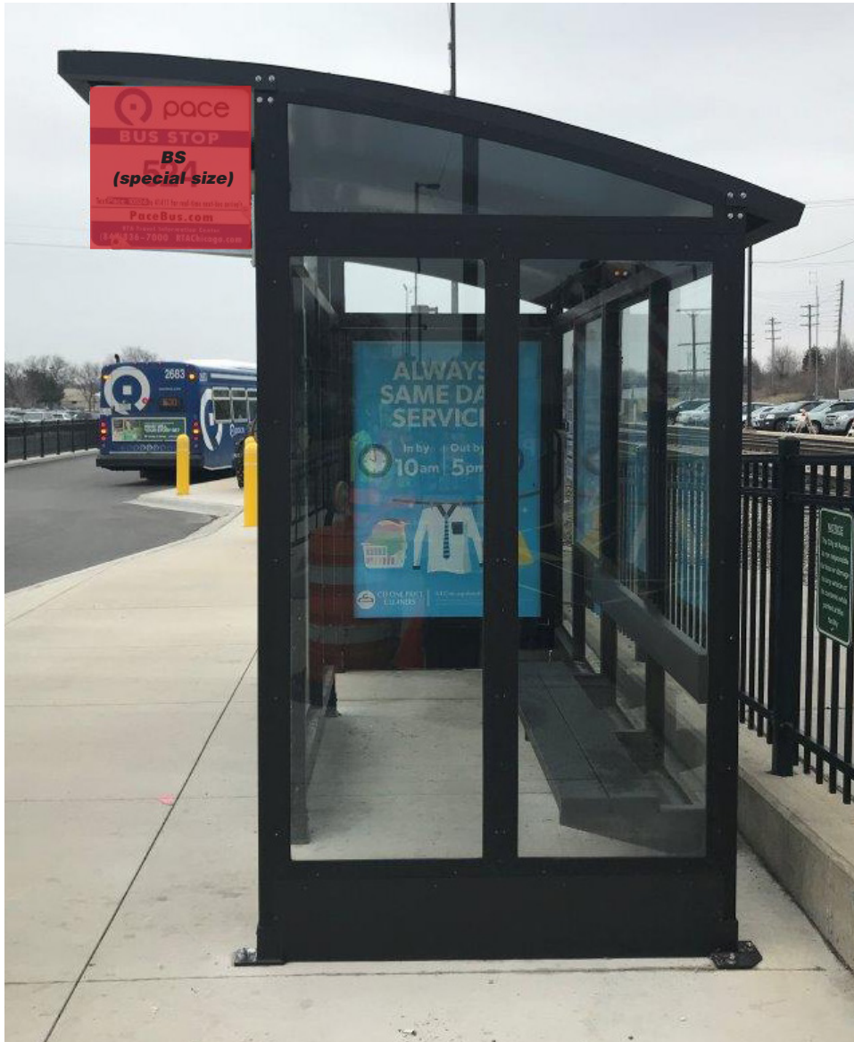
New sign panel replaces existing Pace sign. Reuse existing mounting hardware.
