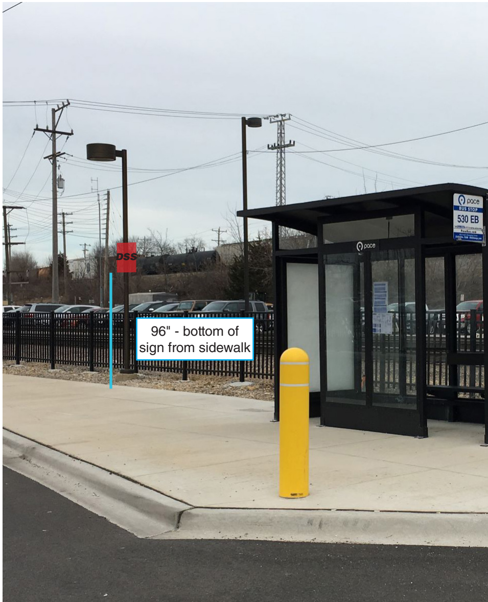
New sign panel mounts to existing light post (center-mount sign panel).
