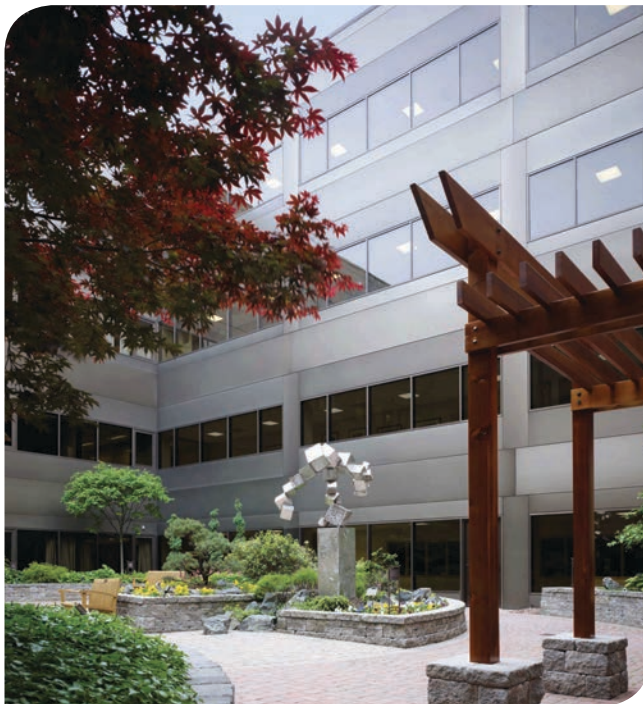
The Blodgett Hospital chiller plant includes free cooling during cold weather and an energy-saving ice storage system.
