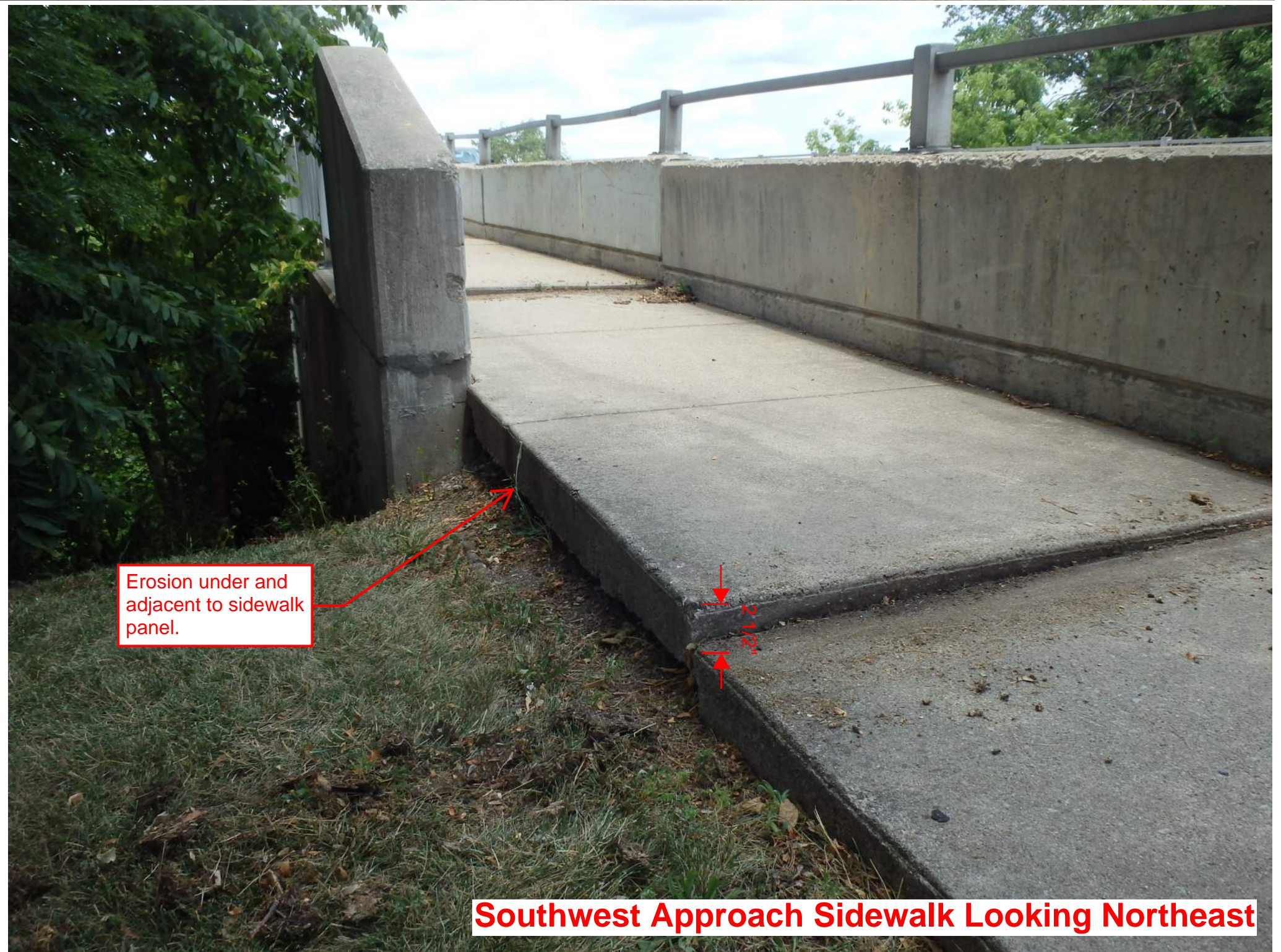
Exhibit A: Remove & replace the first three sidewalk panels south of the S. Approach Slab shown above in the SW quadrant of bridge. At the same time, strengthen the embankment at the end of the retaining wall adjacent to said sidewalk to avoid future erosion at this low spot.
