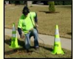
Step 1. Leak Detection
