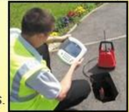
Step 2. Leak Pinpointing
