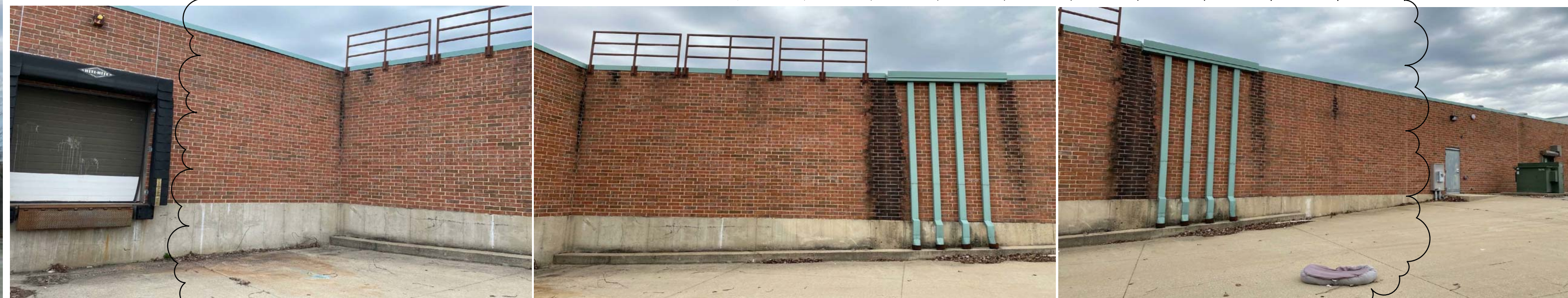
3 EXISTING REAR PHOTOS 1/8" = 1'-0"
