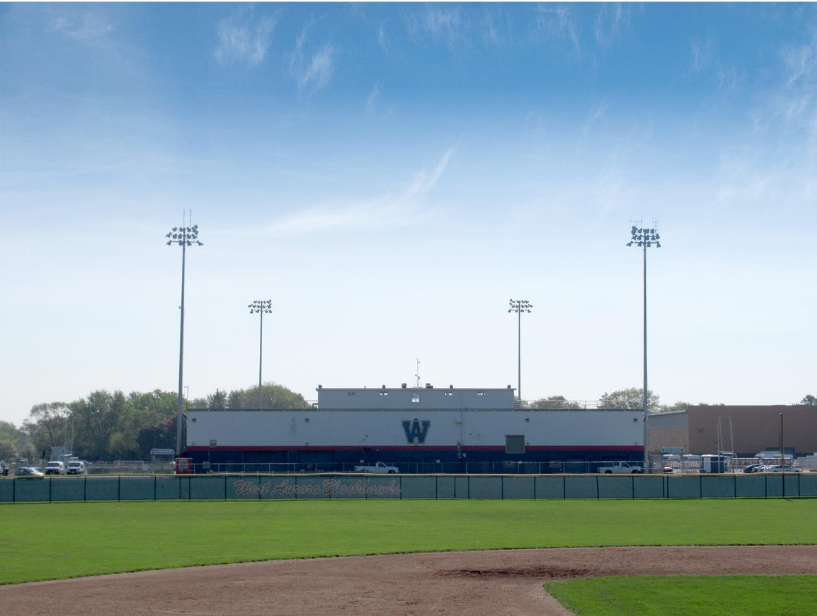
West View (looking East) of (4) Existing Stadium Light Poles
