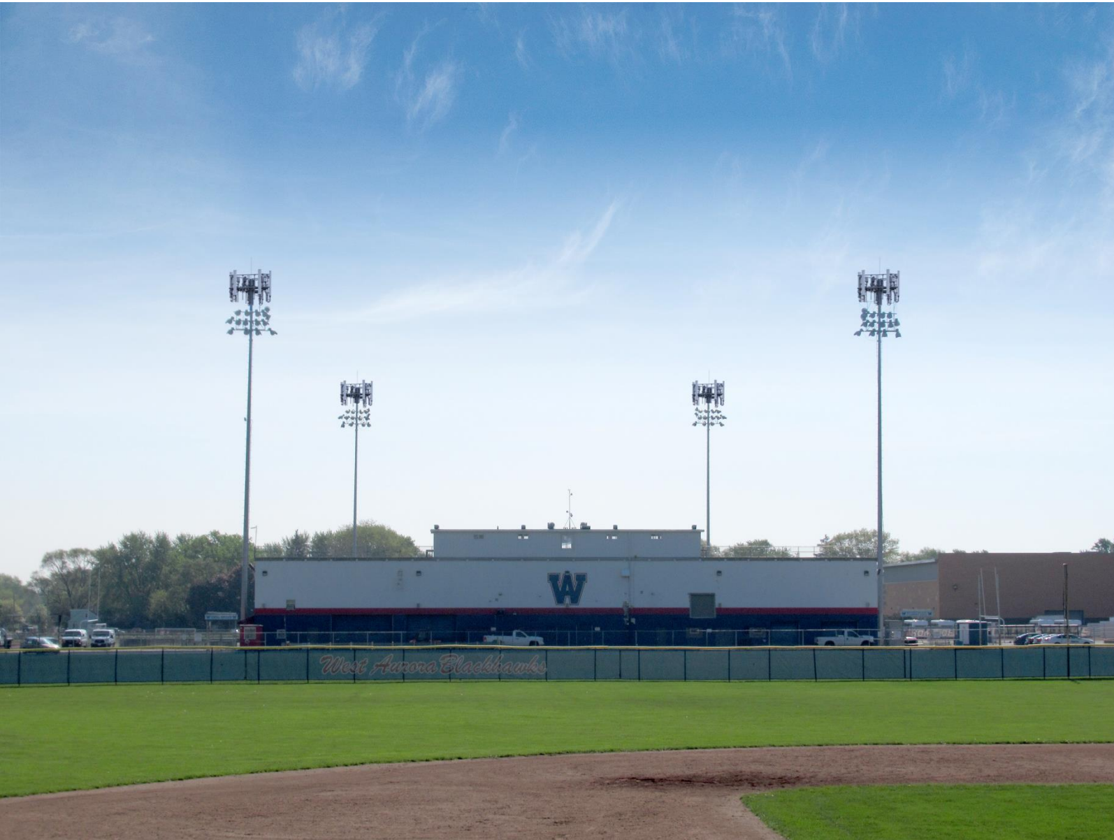
West View (looking East) of (4) Replacement Stadium Light Poles with Carrier Antennas
