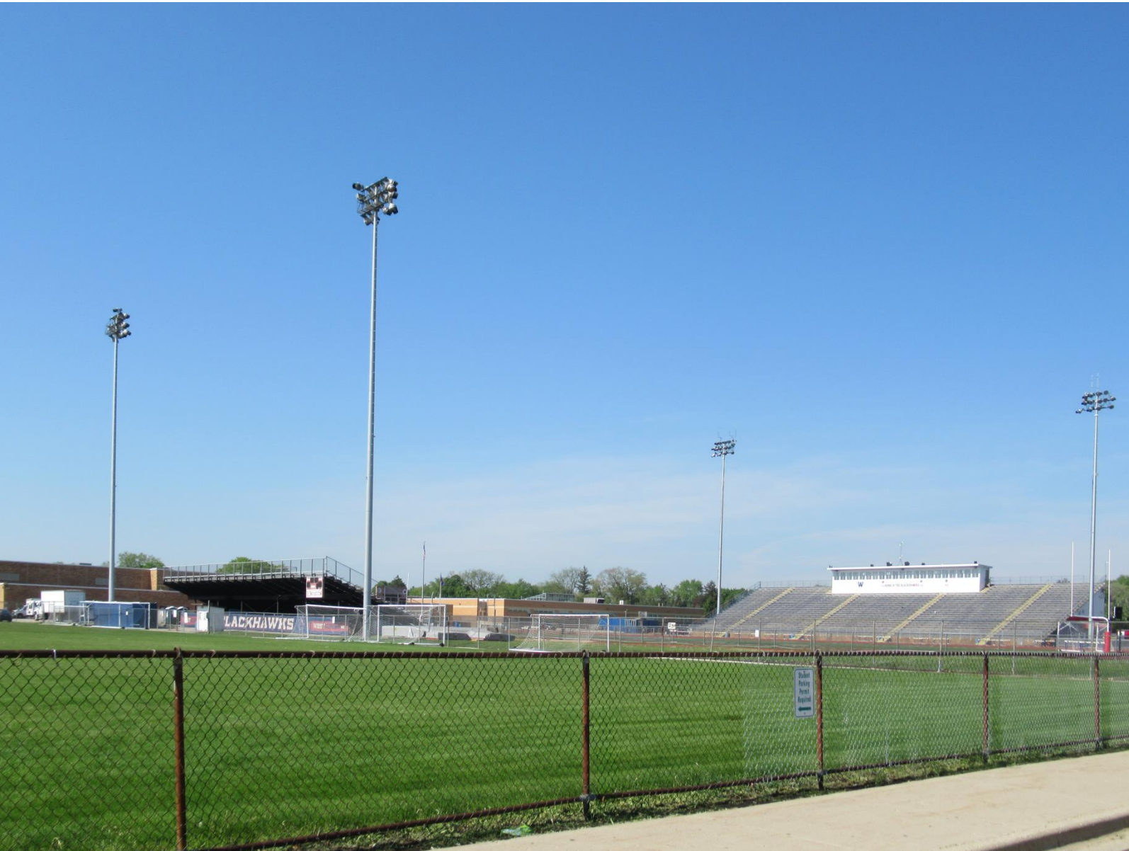
Northeast View (looking Southwest) of (4) Existing Stadium Light Poles
