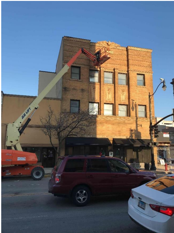
Figure 7. Inspection of east facade on February 22, 2019 (photo courtesy of FHP)
