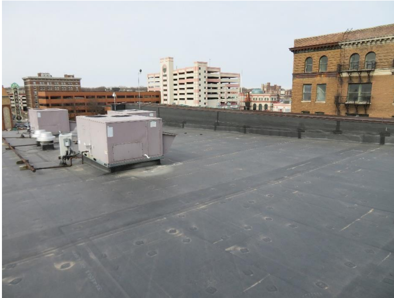
Figure 21. Overall photo of the roof looking northwest
