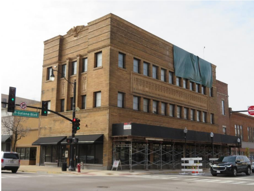
Figure 1. Overall view of the building from the northeast
