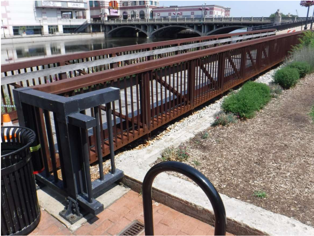
Photo 1 – General Elevation, Looking Northwest
