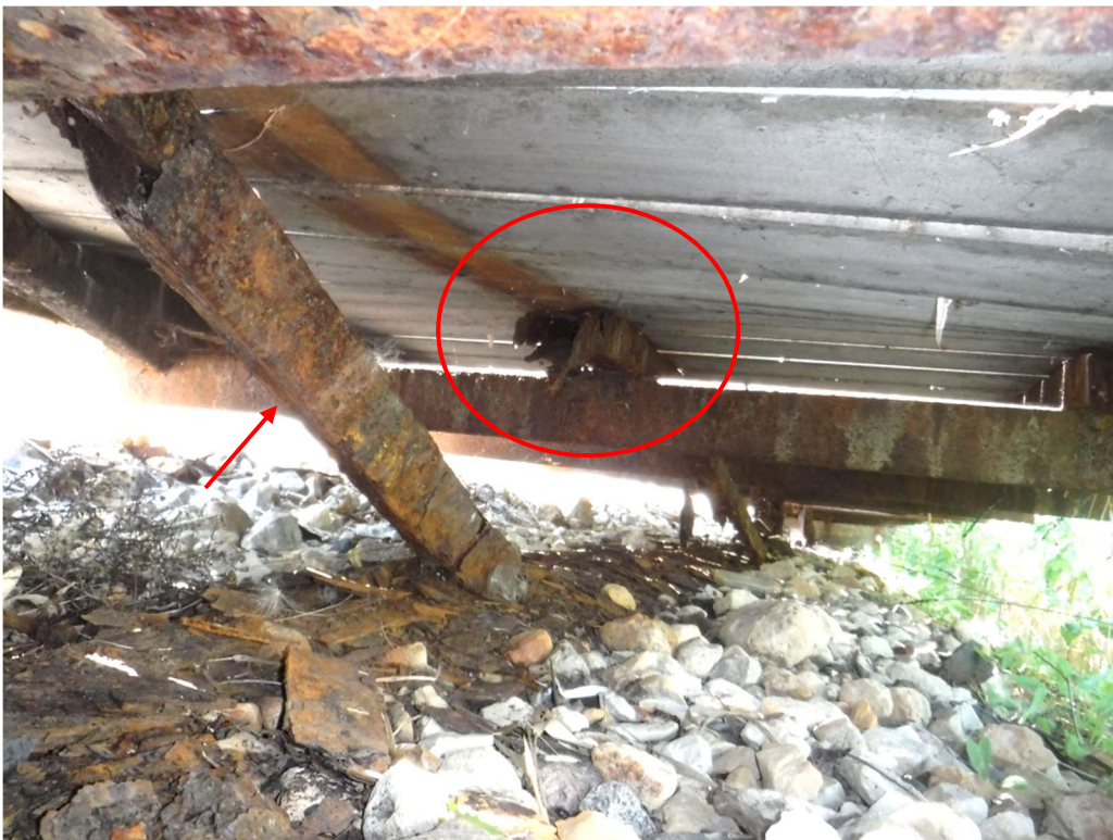
Photo 8 – Typical Center Nailer, Looking South
