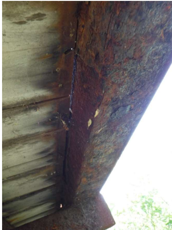
Photo 6 – Bottom Chord Inside and Bottom Faces
