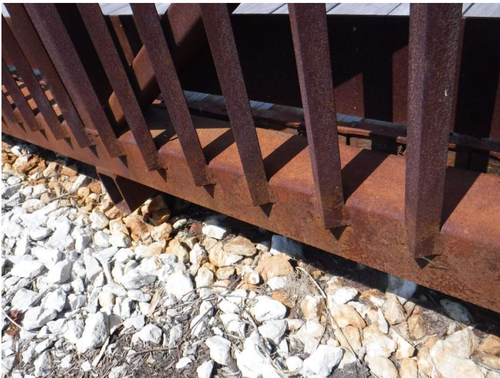
Photo 4 – Top and Outside Faces of Bottom Chord, Looking Down
