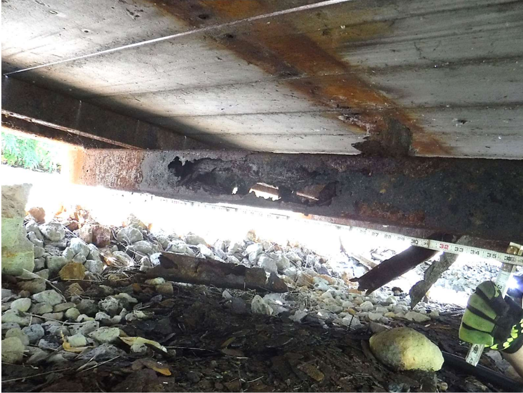
Photo 5 – Floorbeam 5, Looking Southeast
