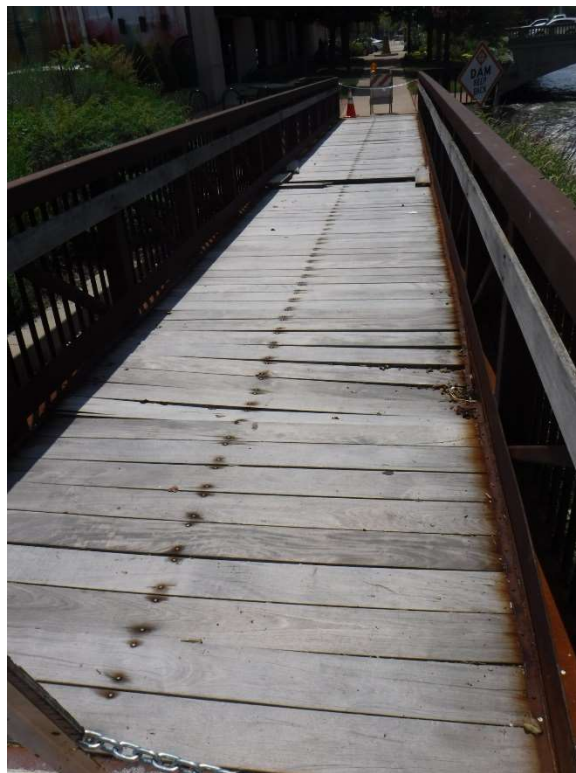
Photo 2 – Top of Deck, Looking South
