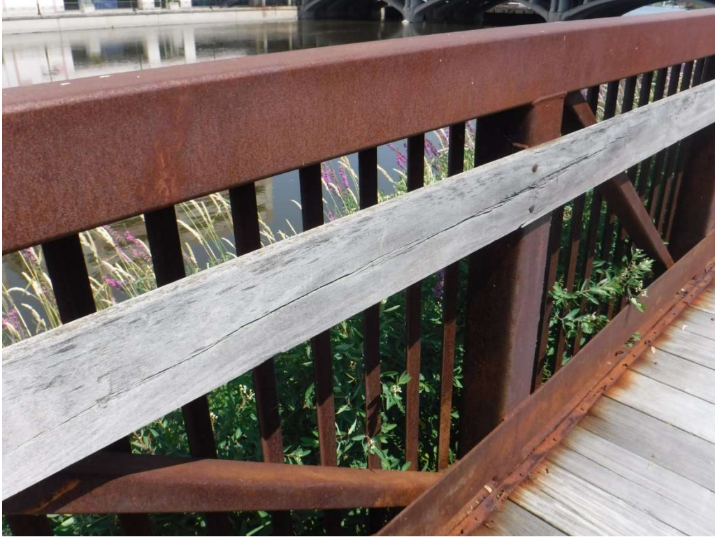
Photo 3 – Typical Truss above Deck and Rub Rail, Looking Northwest
