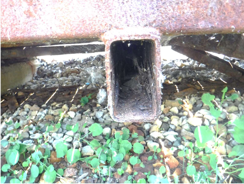
Photo 7 – Typical Inside of Floorbeam
