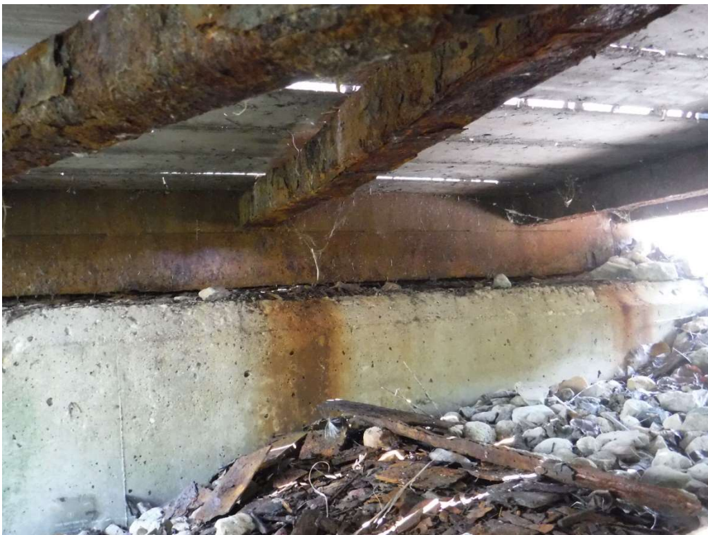
Photo 10 – North Abutment, Looking North
