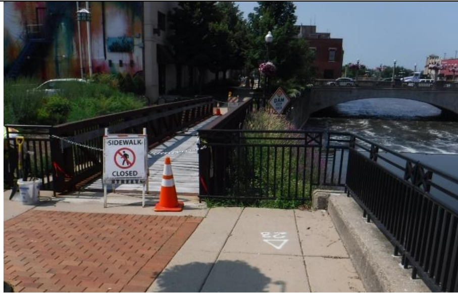
Aurora Riverwalk - Existing View Looking South at Pedestrian Walkway Bridge
