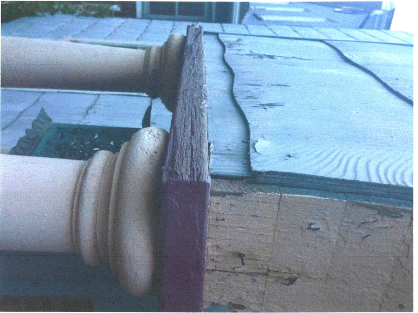
Detail of Siding to Be removed and wood to be Restored
