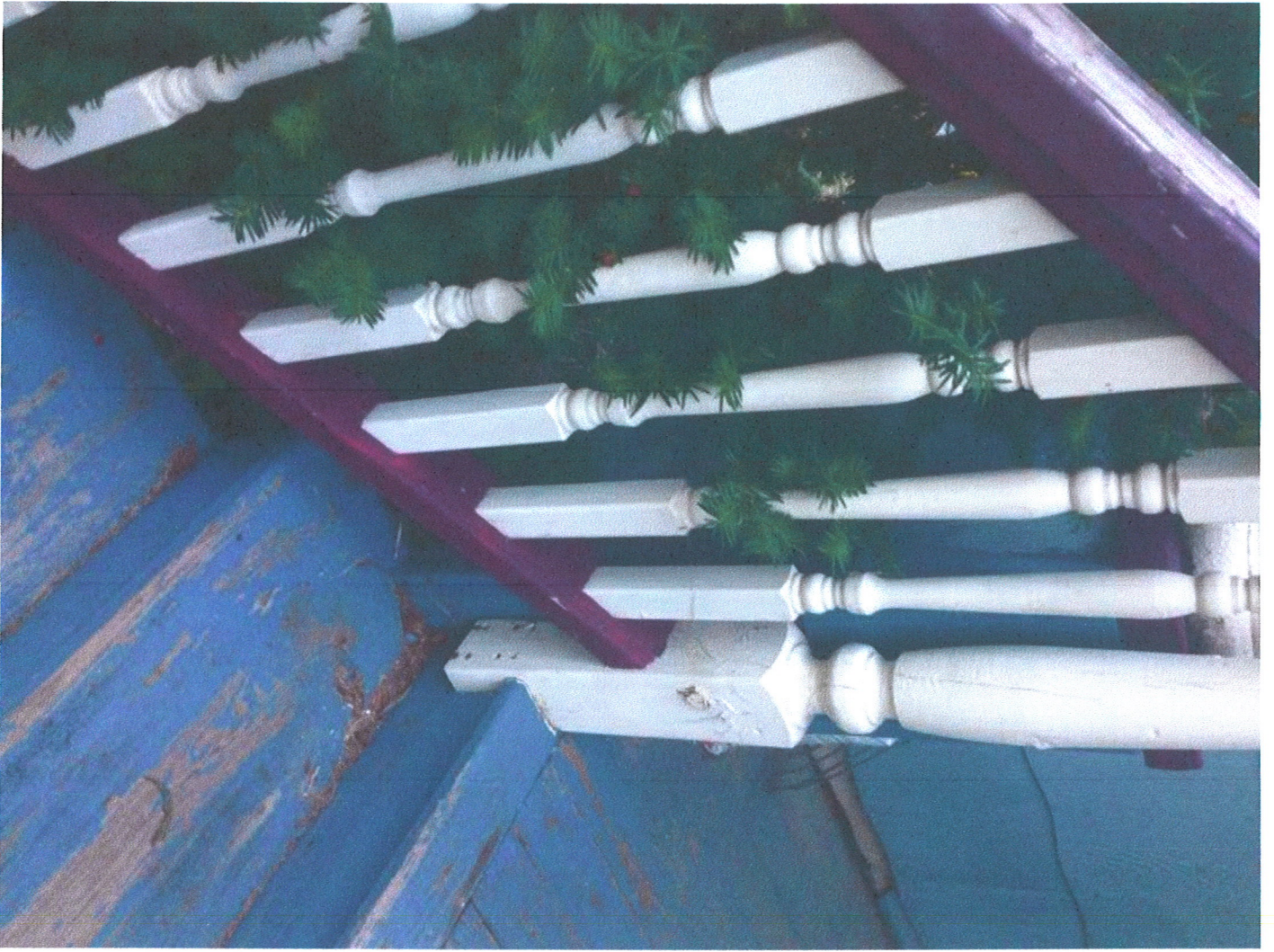
Detail of Porch Condition
