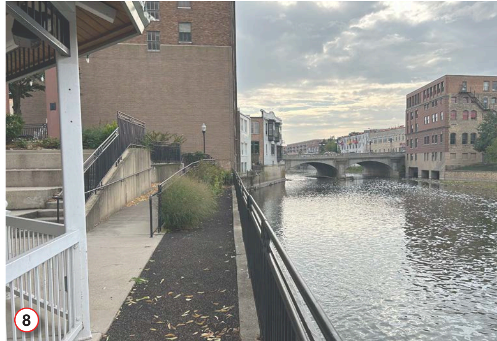
8 Limited space along the river edge. Current pavement is a rubberized surface. Existing guardrails are loose and some are zip-tied together.
