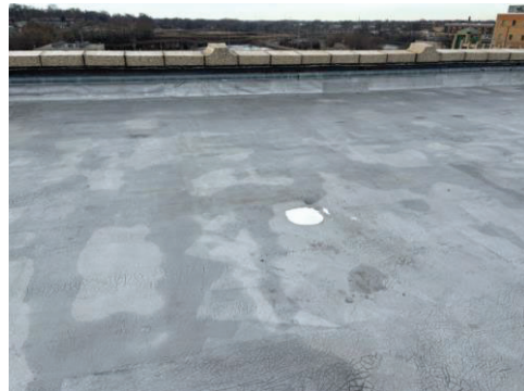
Repairs Completed 44 E. Downers
