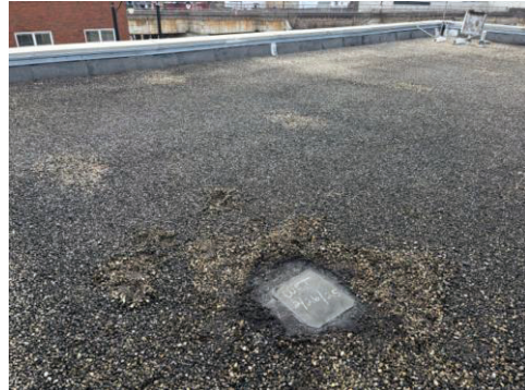
Repairs Completed 77 S. Broadway
