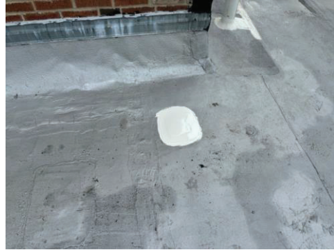
Repairs Completed 44 E. Downers
