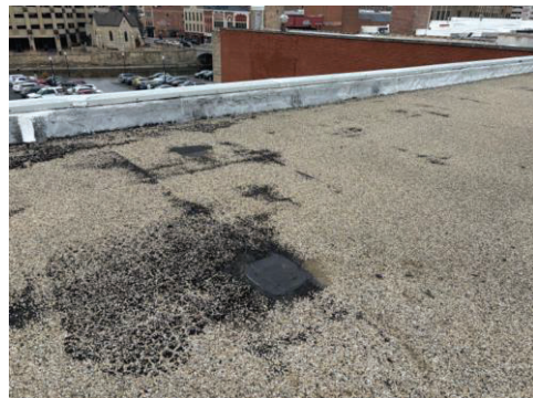
Repairs Completed 77 S Broadway (North section)
