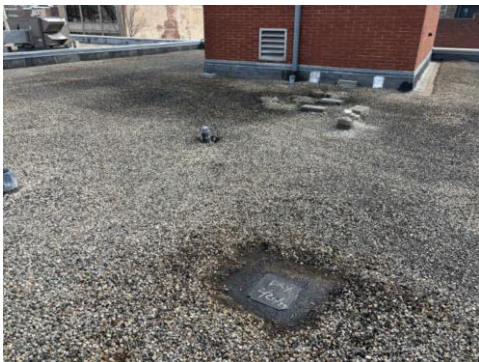
Repairs Completed 77 S. Broadway
