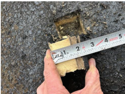
Overview of Roof 77 S Broadway (north section)
