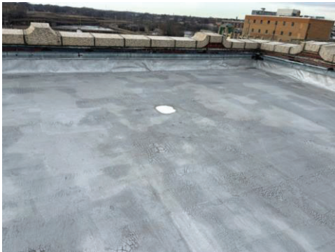
Repairs Completed 44 E. Downers
