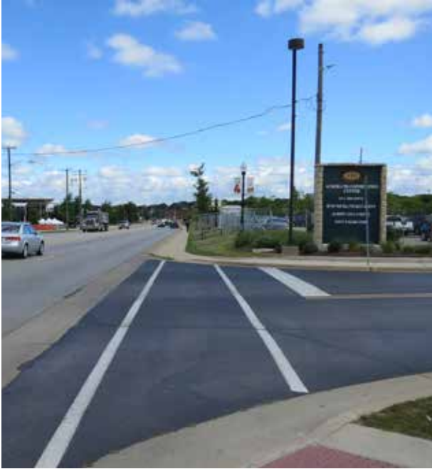
Large curb radii allow for easier turning movements for buses, but they result in a lengthened crossing distance for pedestrians and encourage drivers to take fast turns.
