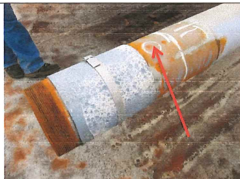
However, the pipe still has some random pitting.
