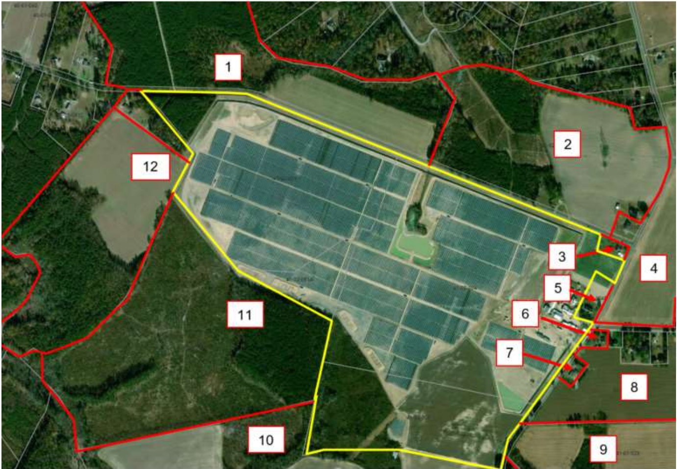
Woodland Solar - Adjoining Properties
