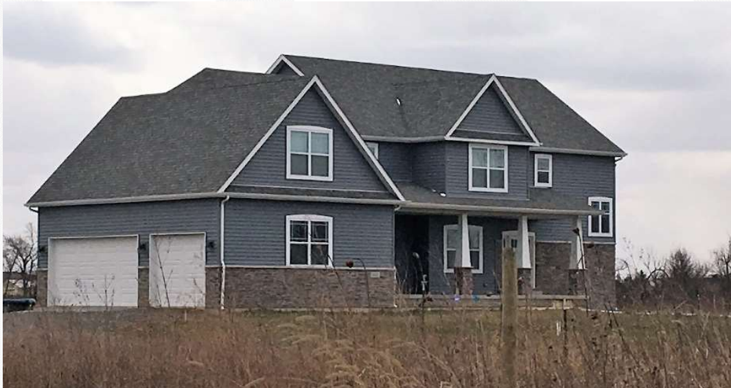
4,255 square foot estate home under construction, adjacent to Portage Solar Farm located in Indiana
