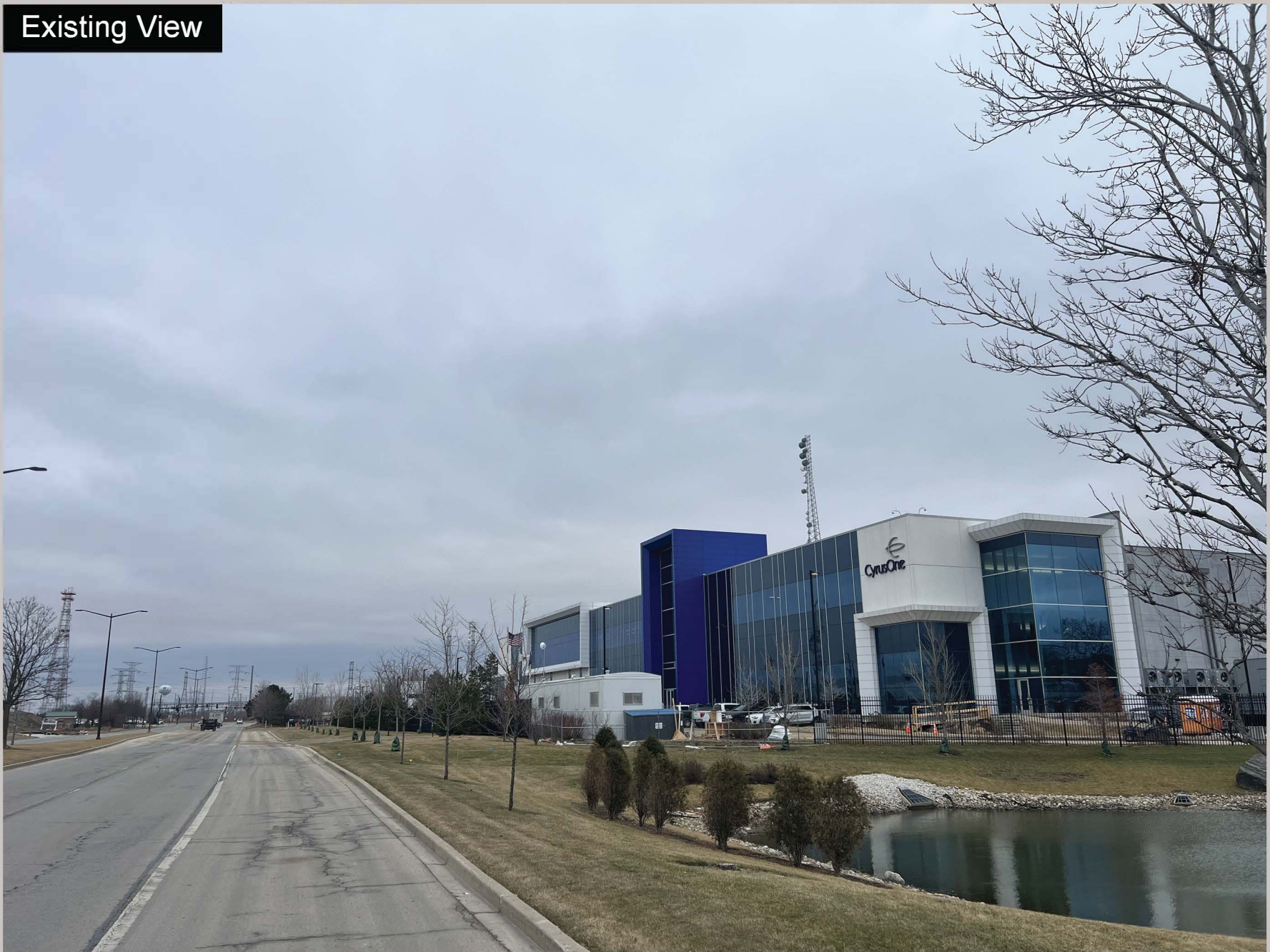
Existing view from location #8 approximately 2,300 feet west of the site.
