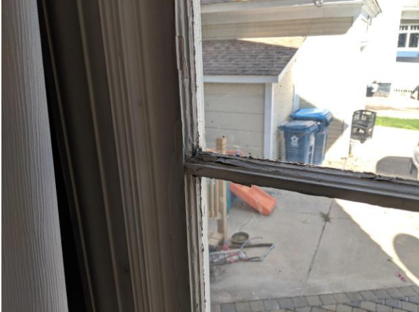
Window 6 (6x5 paned window)
