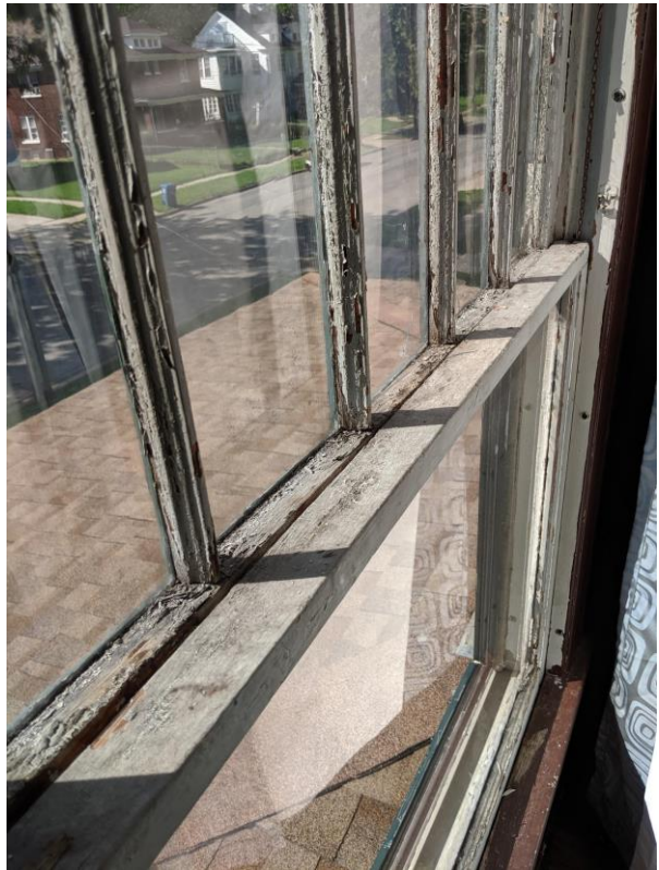
Window 10 West side of house, west facing, 2nd floor
