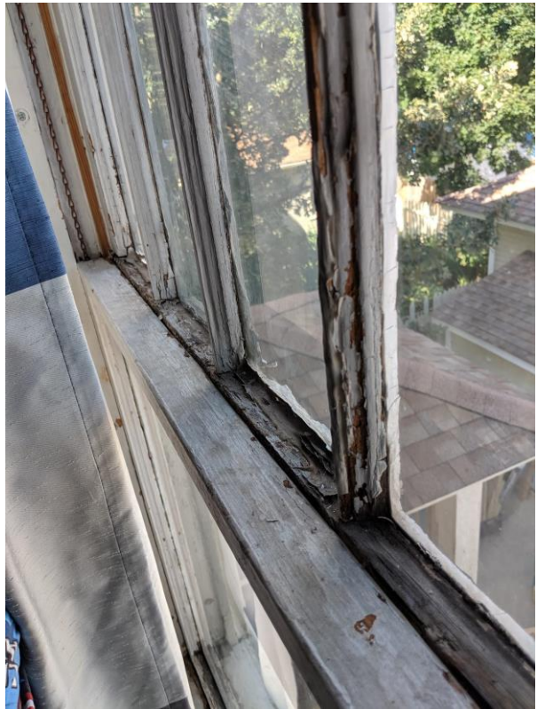
Window 13 East side of house, east facing, 2nd floor
