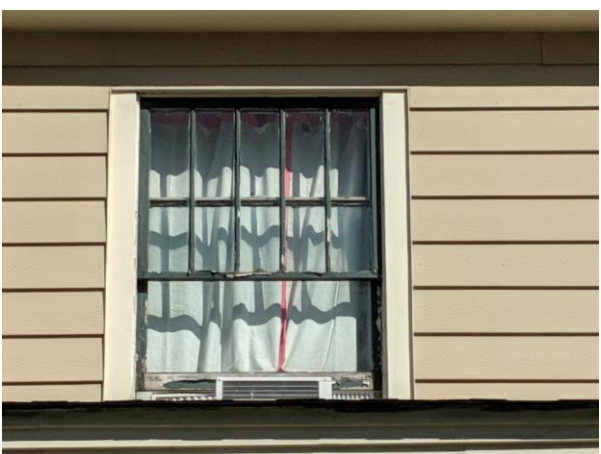
Window 9 (West Facing North most window 2nd Floor)
