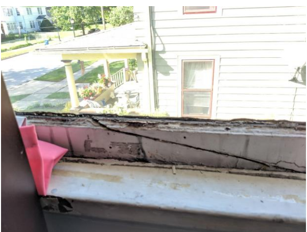
Window 8 (North Facing West Most window 2nd floor)
