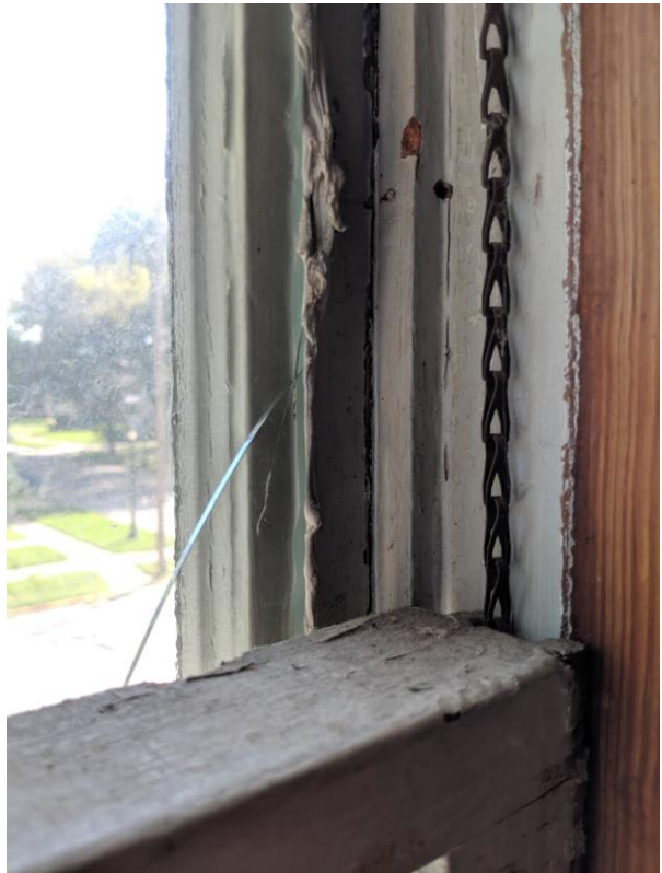
Window 11 south side of house, South facing, 2nd floor
