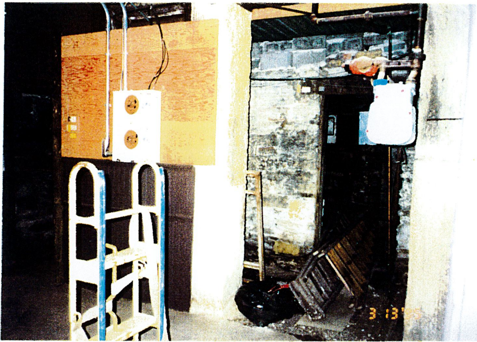
PICTURE 5. Vaulted area in basement.
