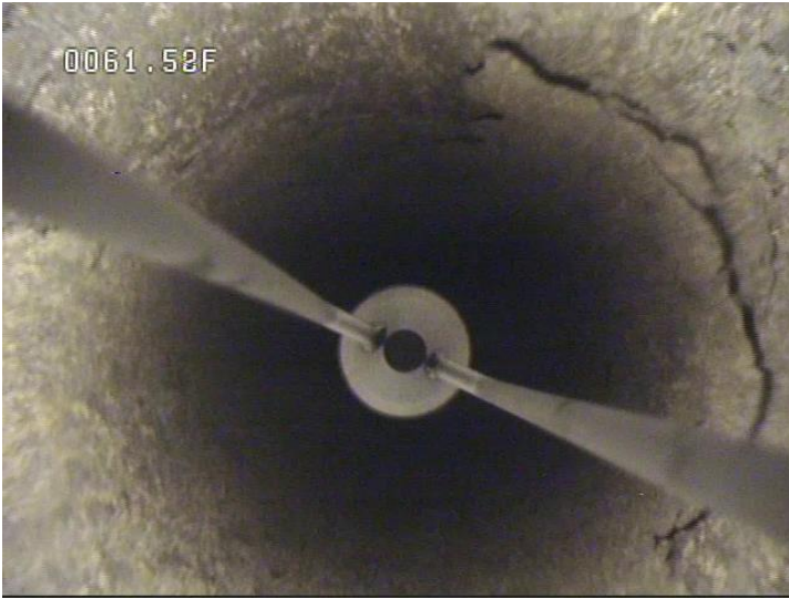
13' - 471' Heavy, large sheets of scale
