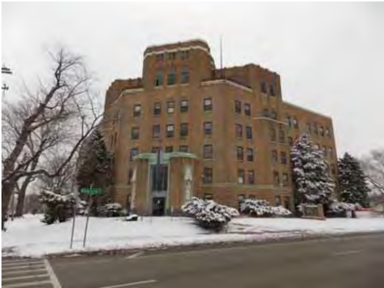
View of the front entrance of the subject building from the intersection of East New York and North 4 th streets
