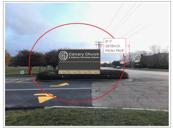
SET A 5" STEEL PIPE IN CONCRETE FOOTING TO BE 3'X4' BY 4' DEEP. CONNECT TO ELECTRICAL SERVICE TO BE PROVIDED BY OTHERS PRIOR TO INSTALL. SEPARATE ELECTRICAL SERVICE FOR EMC UNIT. SEPARATE FOOTING FOR BRICK MASONRY.
