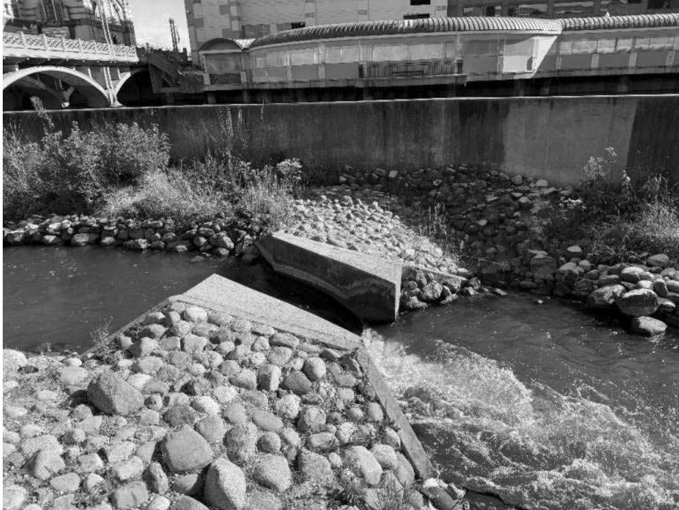
PHOTOGRAPH DS3-1: DROP STRUCTURE 3 (DS3) OVERALL VIEW
