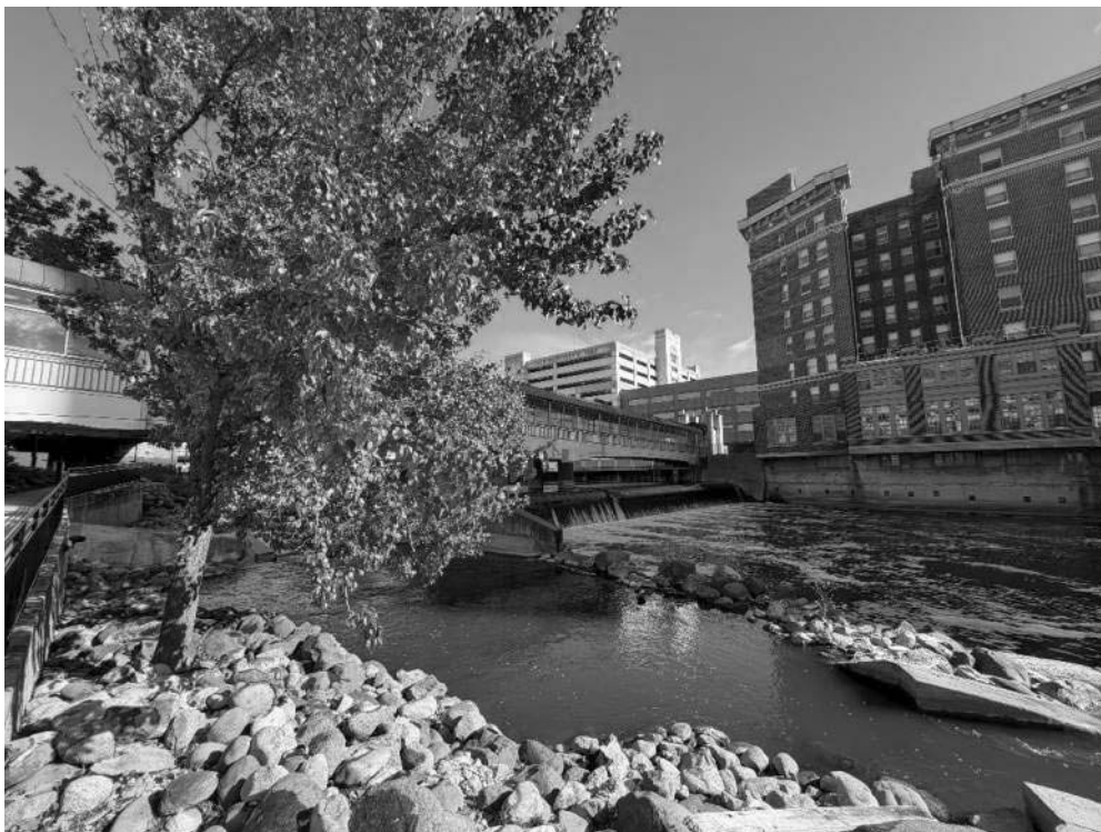
PHOTOGRAPH OUT-2: OUTLET STRUCTURE LOOKING UPSTREAM
