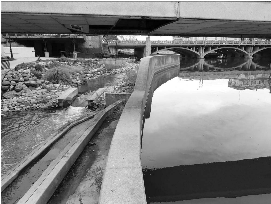
Photograph 6. View of the Canoe Chute East Wall, Looking North.
