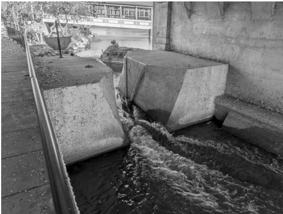
PHOTOGRAPH DS1-2: DOWNSTREAM SIDE OF DS1
