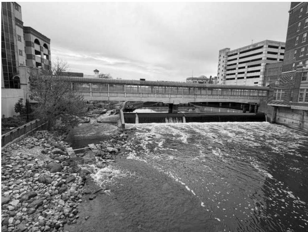
PHOTOGRAPH WD-1: WEST DAM OVERALL VIEW – LOOKING AT DOWNSTREAM SIDE
