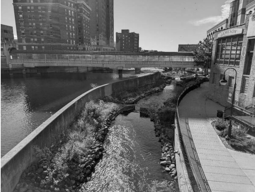
FIGURE 1 – FOX RIVER AND CANOE CHUTE UPSTREAM OF WEST DAM
