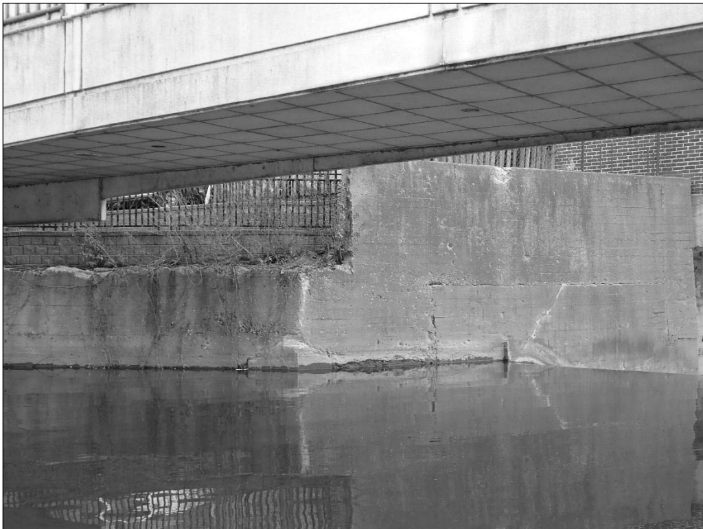
Photograph 18. View of the East Abutment, Looking East.
