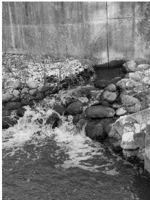
PHOTOGRAPH DS4-2: FLOW THROUGH CANOE CHUTE EAST WALL UPSTREAM OF DS4
