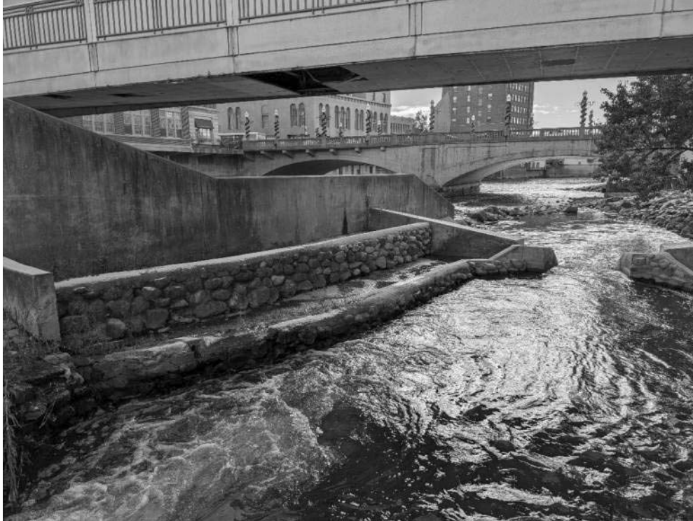
PHOTOGRAPH DS5-1: DROP STRUCTURE 5 (DS5) UPSTREAM VIEW
