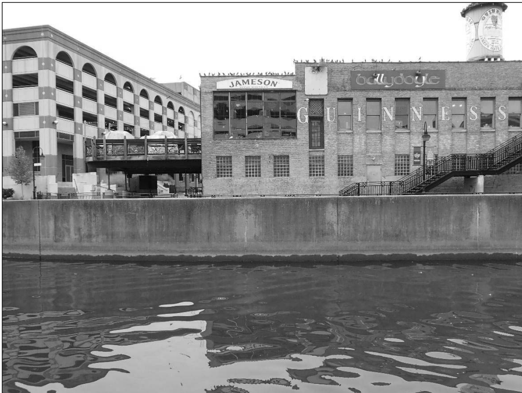
Photograph 8. View of the Canoe Chute East Wall from Station 0+50 to Station 0+75, Looking West.
