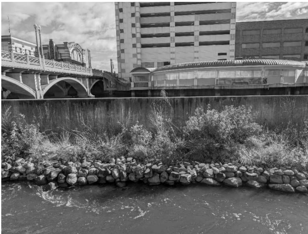
PHOTOGRAPH DS2-4: TYPICAL CANOE CHUTE EAST WALL SECTION
