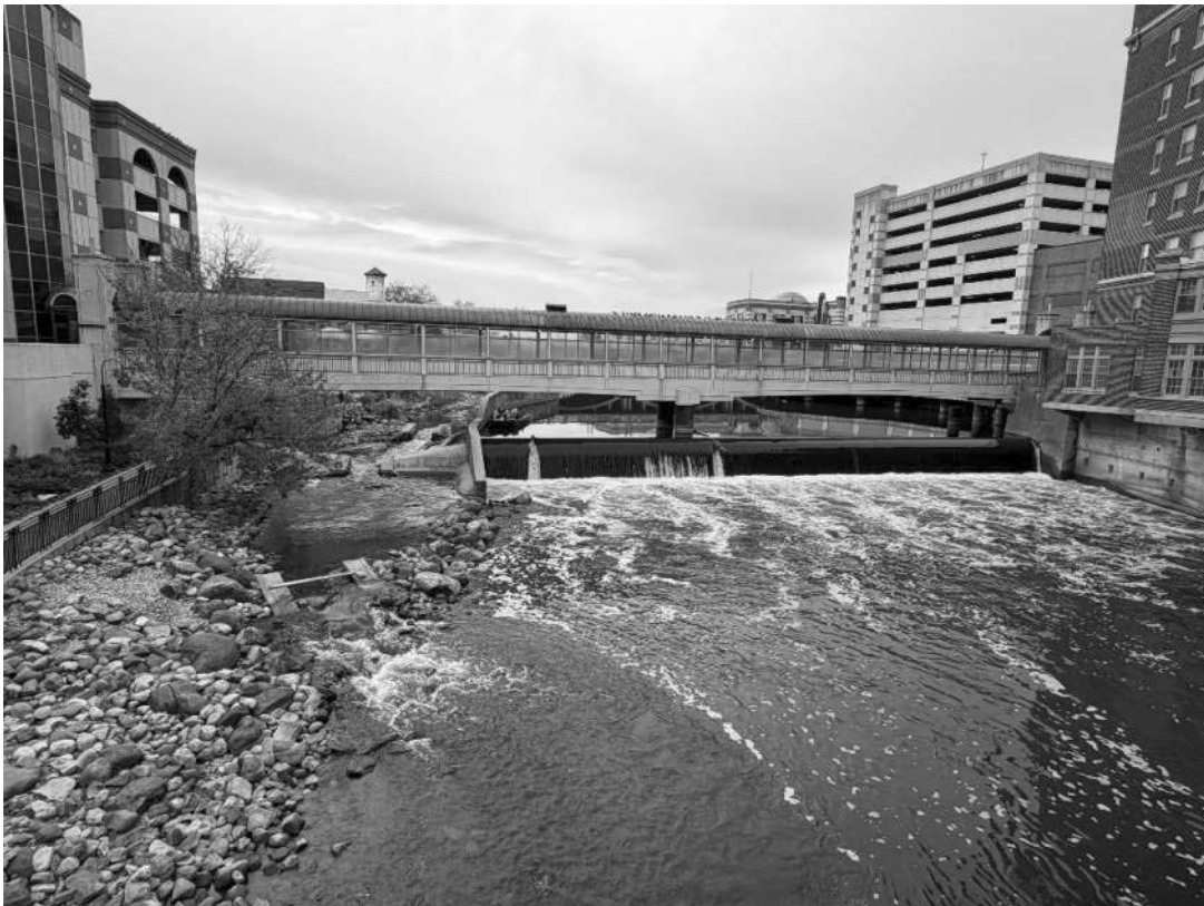
FIGURE 8 – WEST DAM AND CANOE CHUTE LOOKING UPSTREAM
