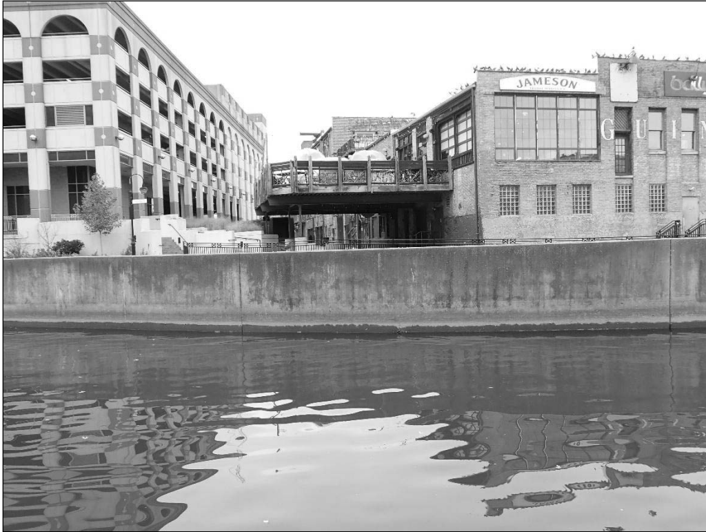
Photograph 9. View of the Canoe Chute East Wall from Station 0+75 to Station 1+25, Looking West.
