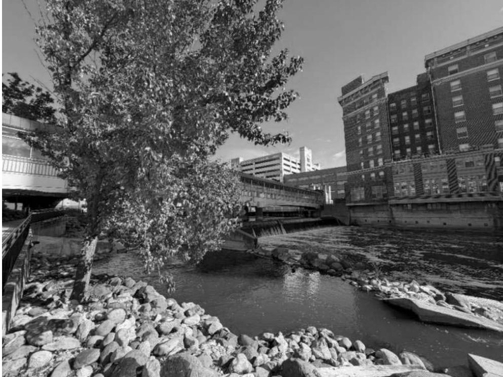
PHOTOGRAPH CC-3: CANOE CHUTE OUTLET OVERALL VIEW – LOOKING DOWNSTREAM TO UPSTREAM AT DOWNSTREAM END
