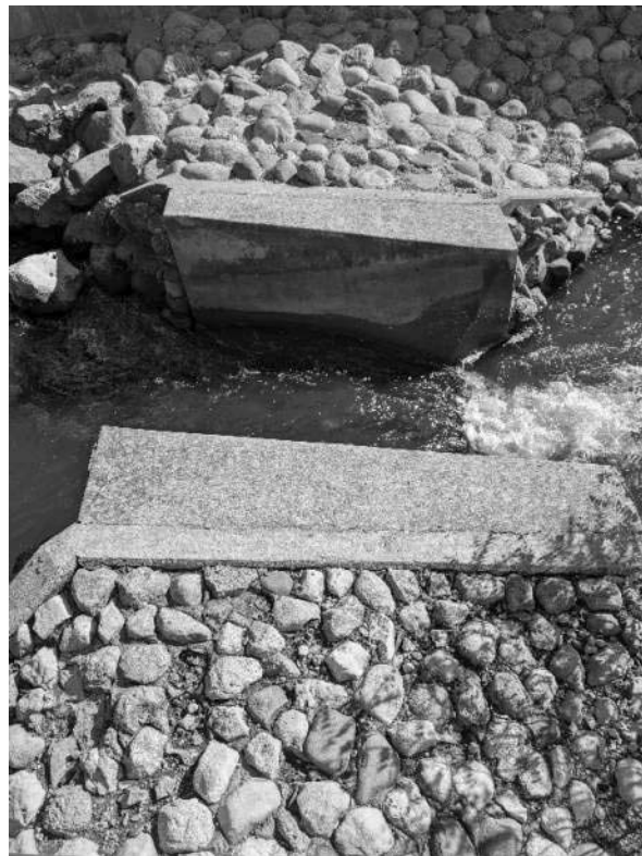
PHOTOGRAPH CC-4: DROP STRUCTURE (TYPICAL)
