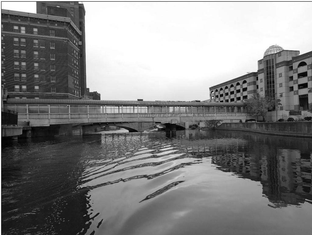
Photograph 2. Overall View of the Aurora Dam, Looking Southwest.
