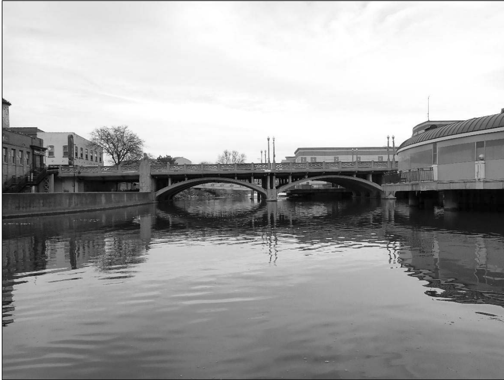
Photograph 3. View of the Upstream Channel, Looking North.
