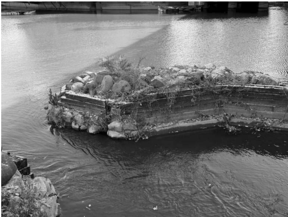
PHOTOGRAPH IN-2: INLET STRUCTURE AND STOP LOG SLOTS
