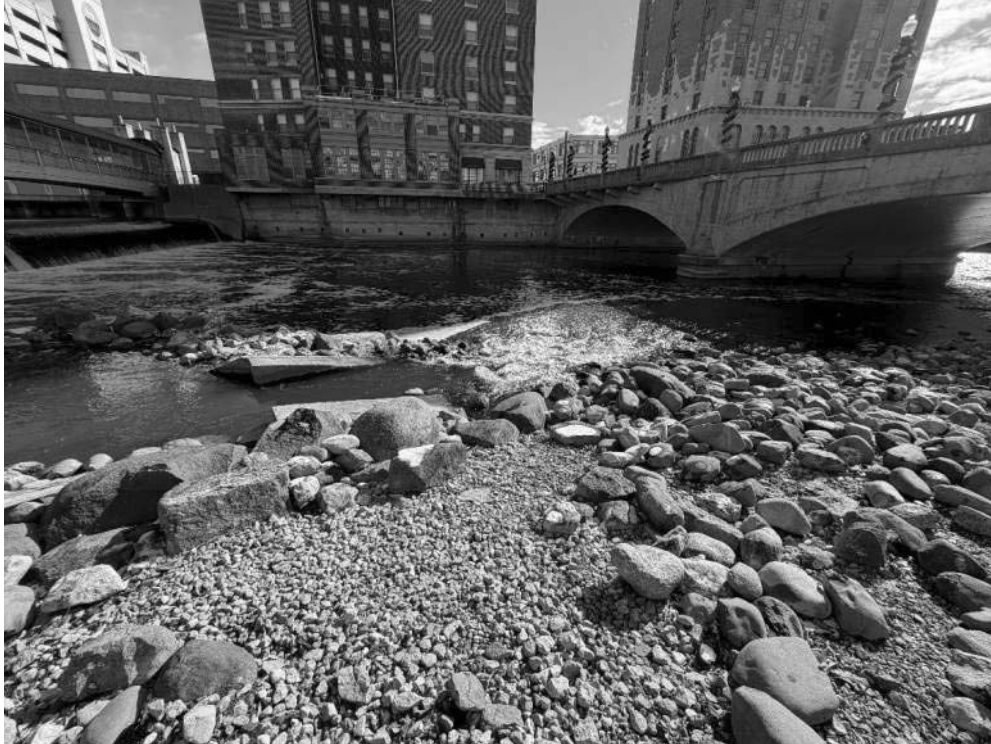
PHOTOGRAPH OUT-1: OUTLET STRUCTURE LOOKING DOWNSTREAM
