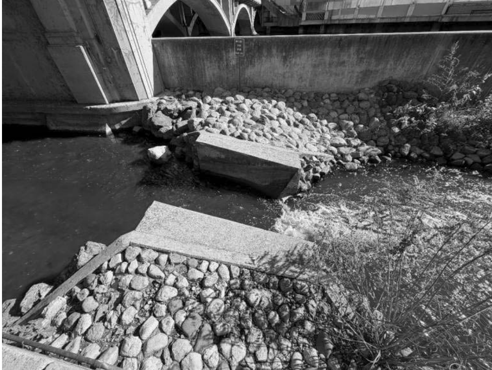
PHOTOGRAPH DS2-1: DROP STRUCTURE 2 (DS2) OVERALL VIEW
