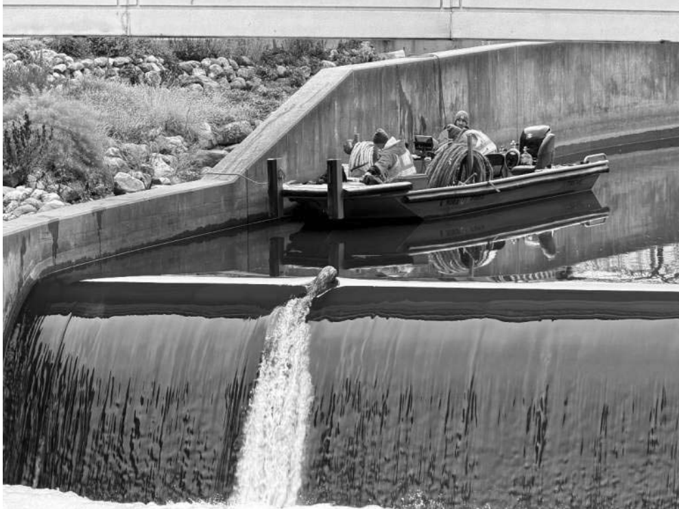
PHOTOGRAPH WD-2: WEST DAM CANOE CHUTE EAST WALL ALONG FOX RIVER
