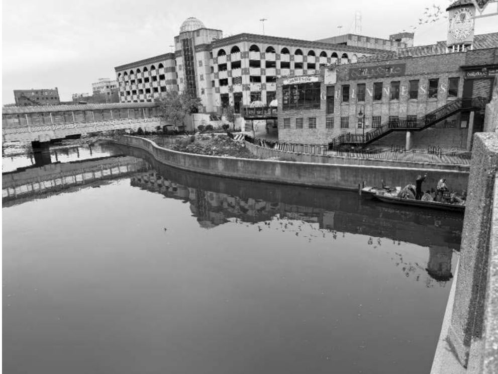
PHOTOGRAPH INSP-1: CANOE CHUTE EAST WALL INSPECTION ALONG FOX RIVER
