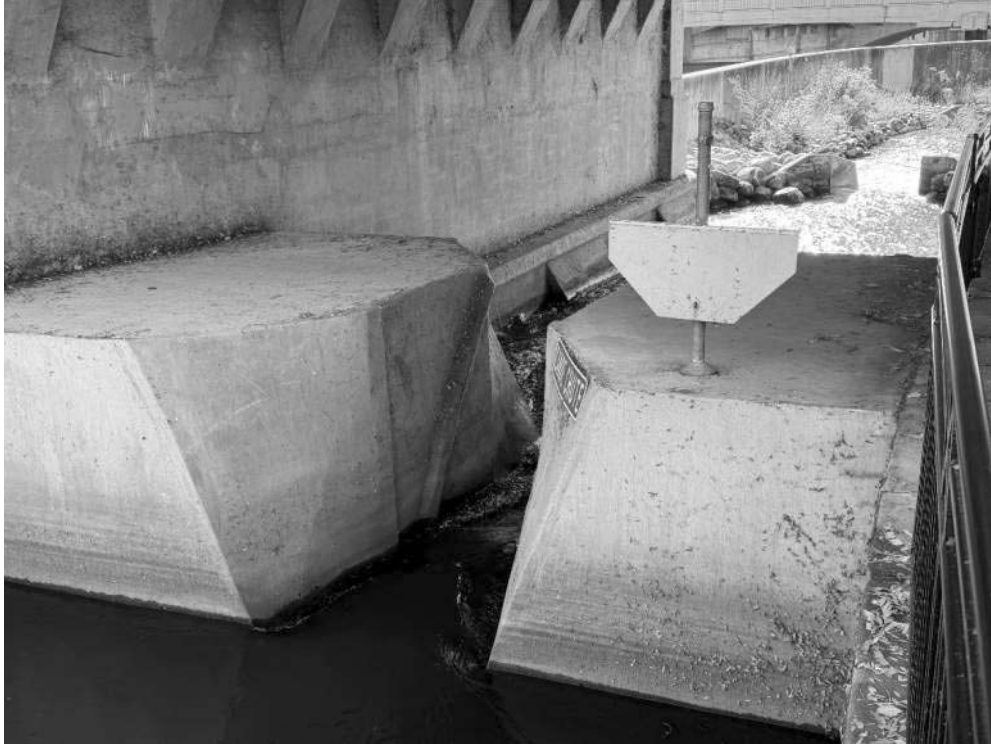
PHOTOGRAPH DS1-1: UPSTREAM FACE OF DROP STRUCTURE 1 (DS1)
