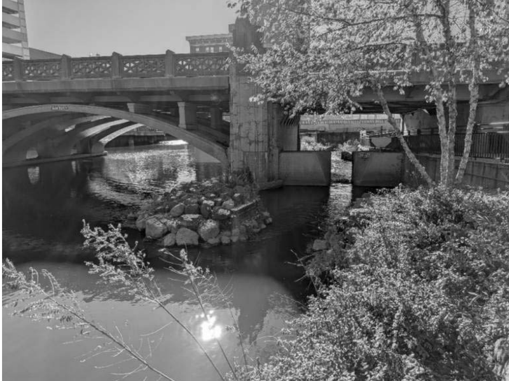
PHOTOGRAPH IN-1: INLET STRUCTURE UPSTREAM SIDE
