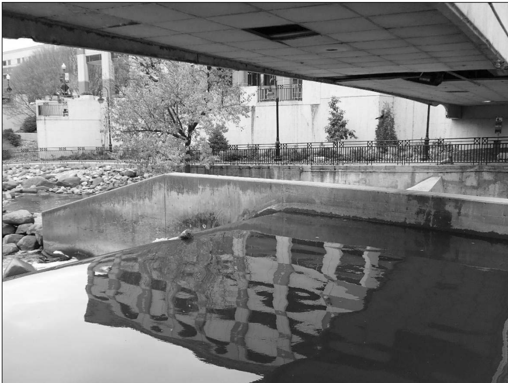
Photograph 12. View of the Canoe Chute East Wall from Station 2+20 to Station 2+62, Looking Southwest.
