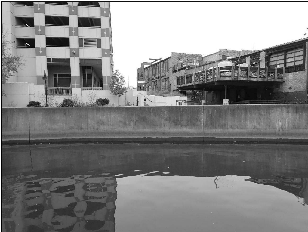
Photograph 10. View of the Canoe Chute East Wall from Station 1+25 to Station 1+75, Looking West.
