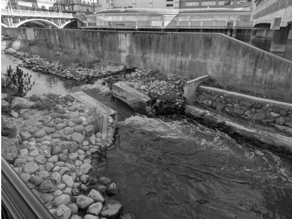
PHOTOGRAPH DS4-5: DS4 DOWNSTREAM VIEW LOOKING UPSTREAM
