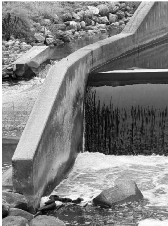
PHOTOGRAPH WD-3: WEST DAM CANOE CHUTE EAST WALL ALONG FOX RIVER)
