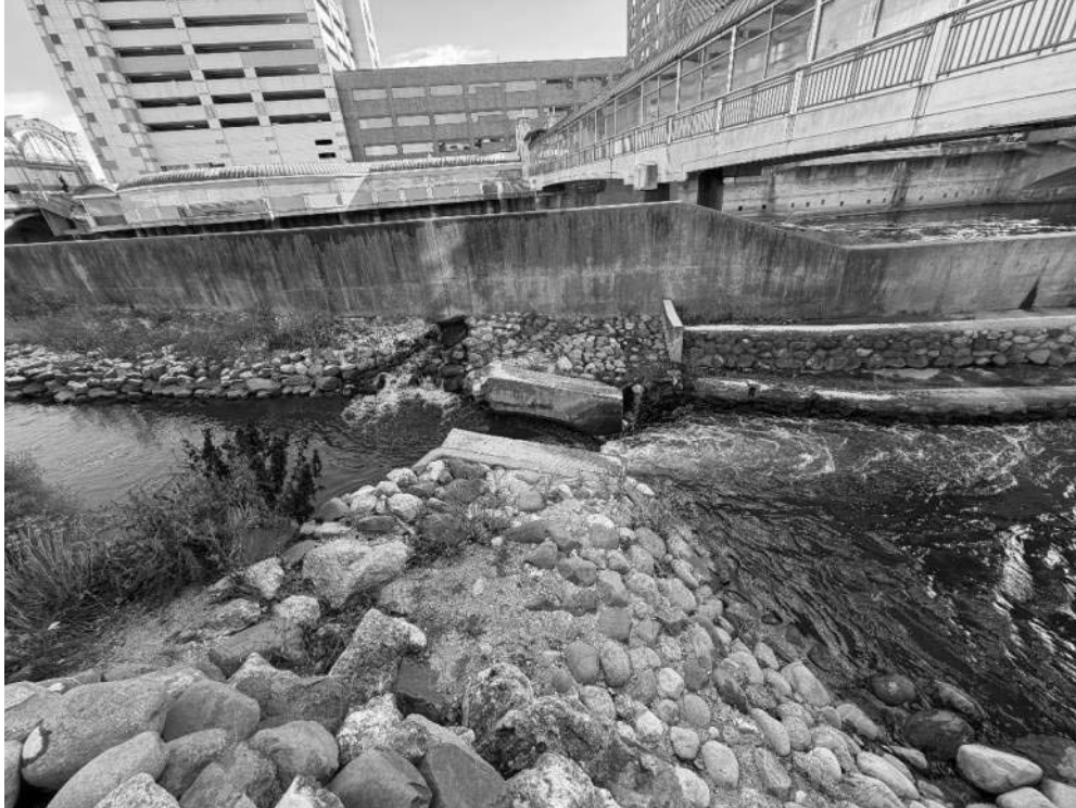
PHOTOGRAPH DS4-1: DROP STRUCTURE 4 (DS4) OVERALL VIEW
