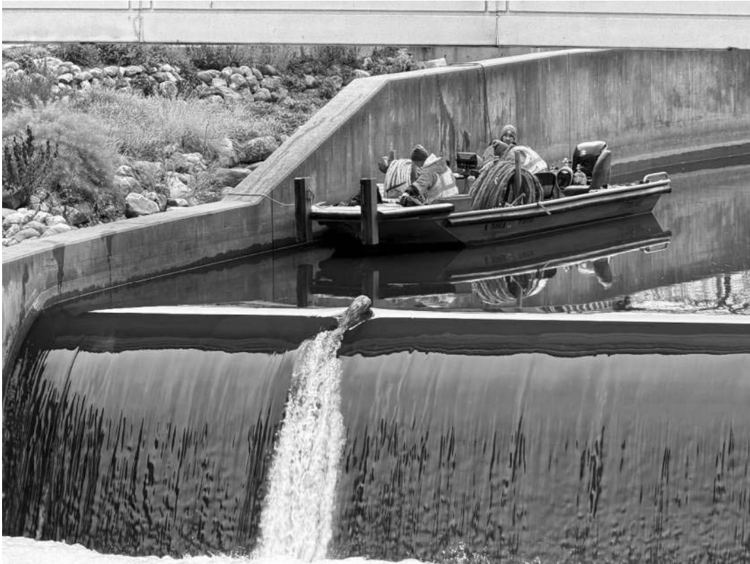
FIGURE 2 – INSPECTION TEAM ALONG CANOE CHUTE EAST WALL
