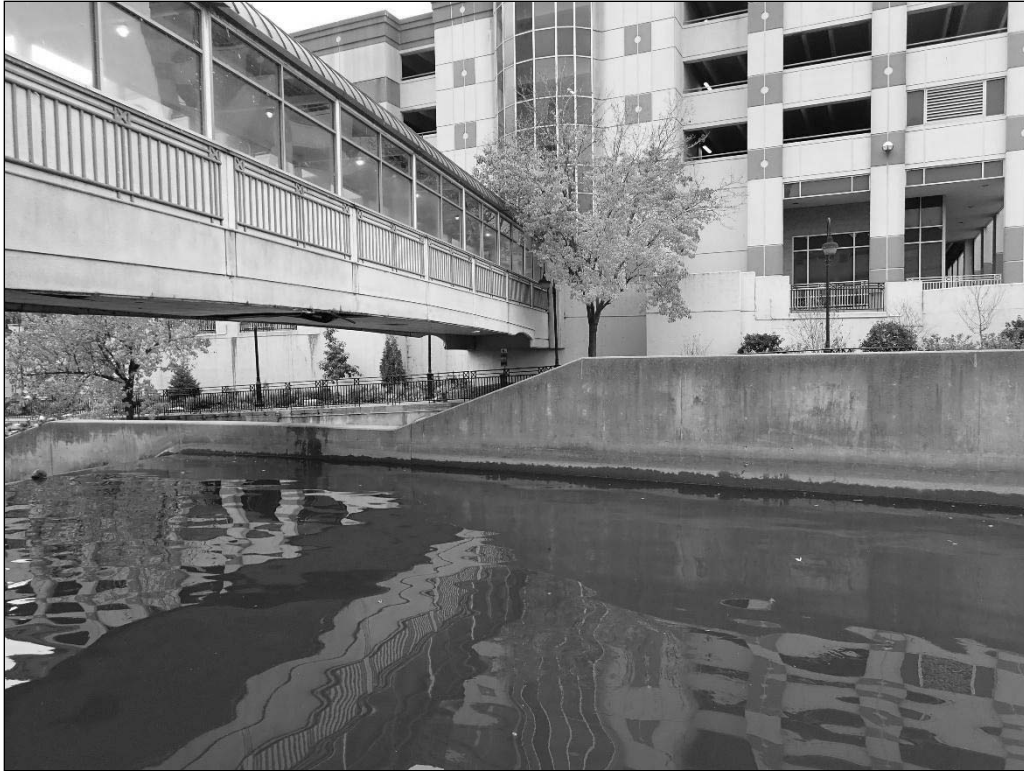
Photograph 11. View of the Canoe Chute East Wall from Station 1+75 to Station 2+35, Looking Southwest.
