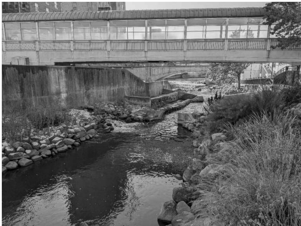
PHOTOGRAPH CC-2: CANOE CHUTE OVERALL VIEW – LOOKING UPSTREAM TO DOWNSTREAM AT DS4
