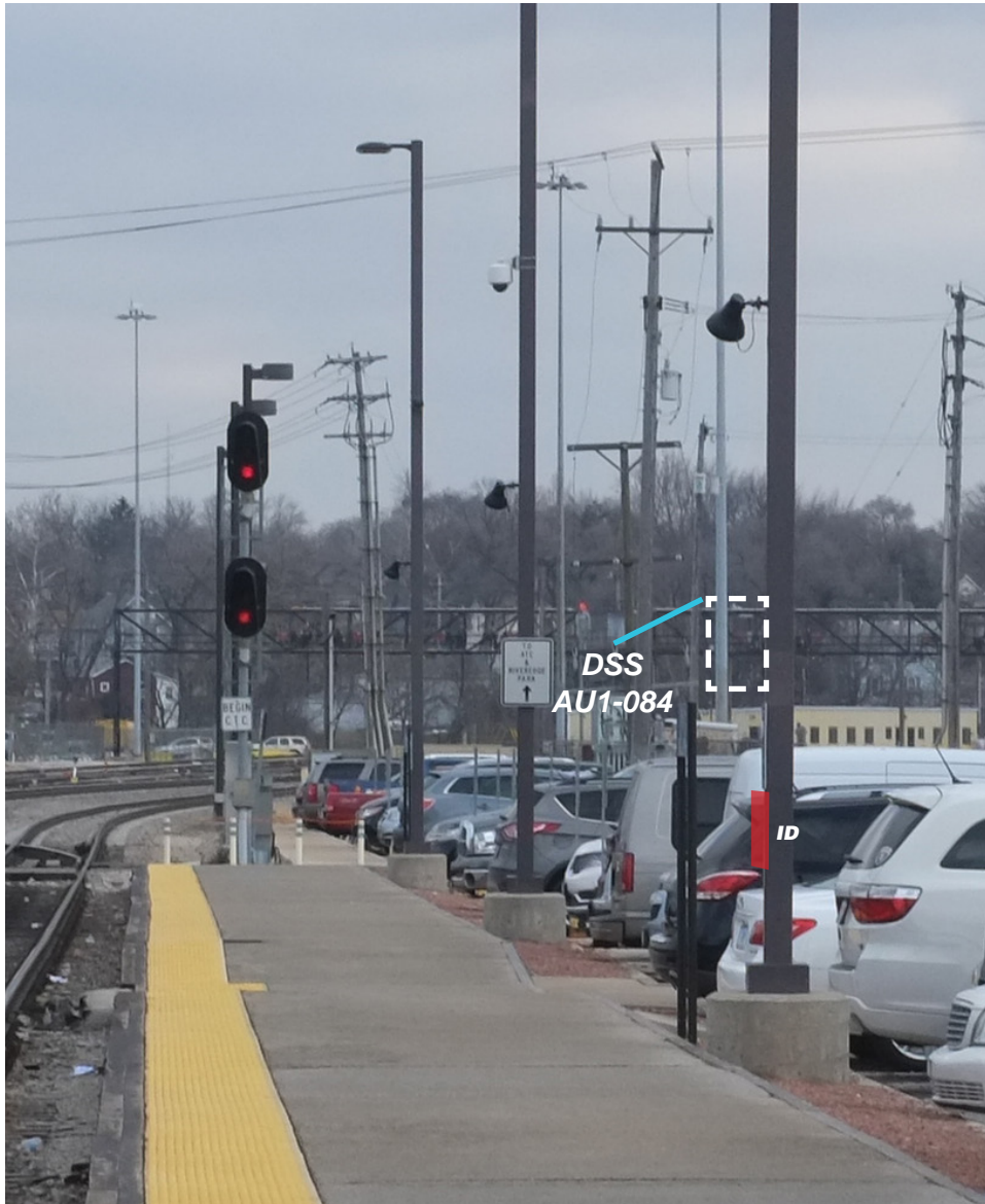
New sign panel mounts to existing light post. Verify mounting height with existing suicide sign.
