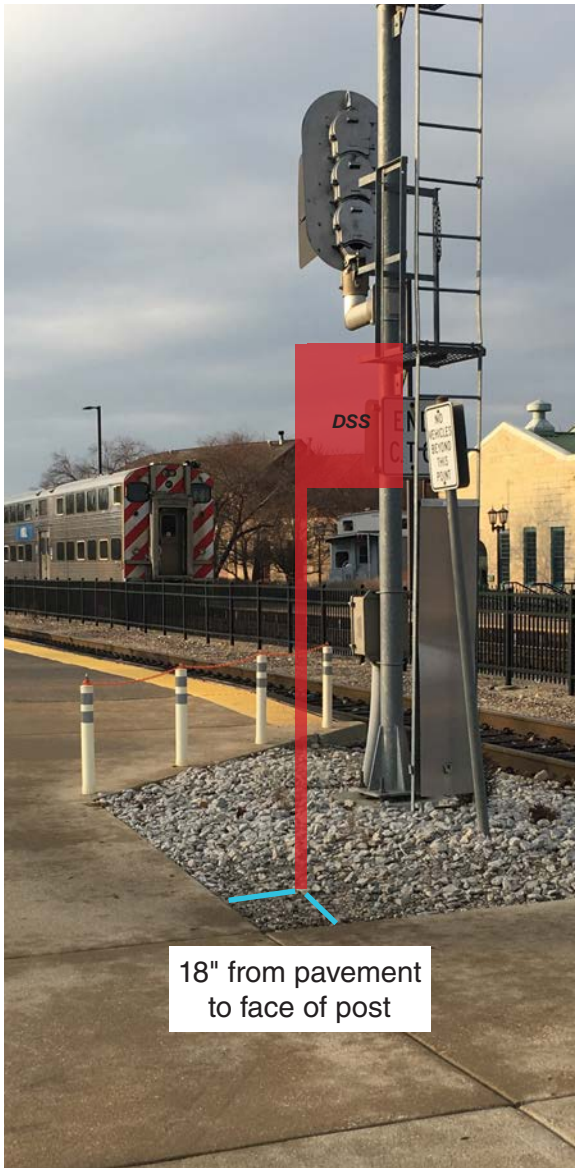
New sign panel and sign post. Direct bury post.
