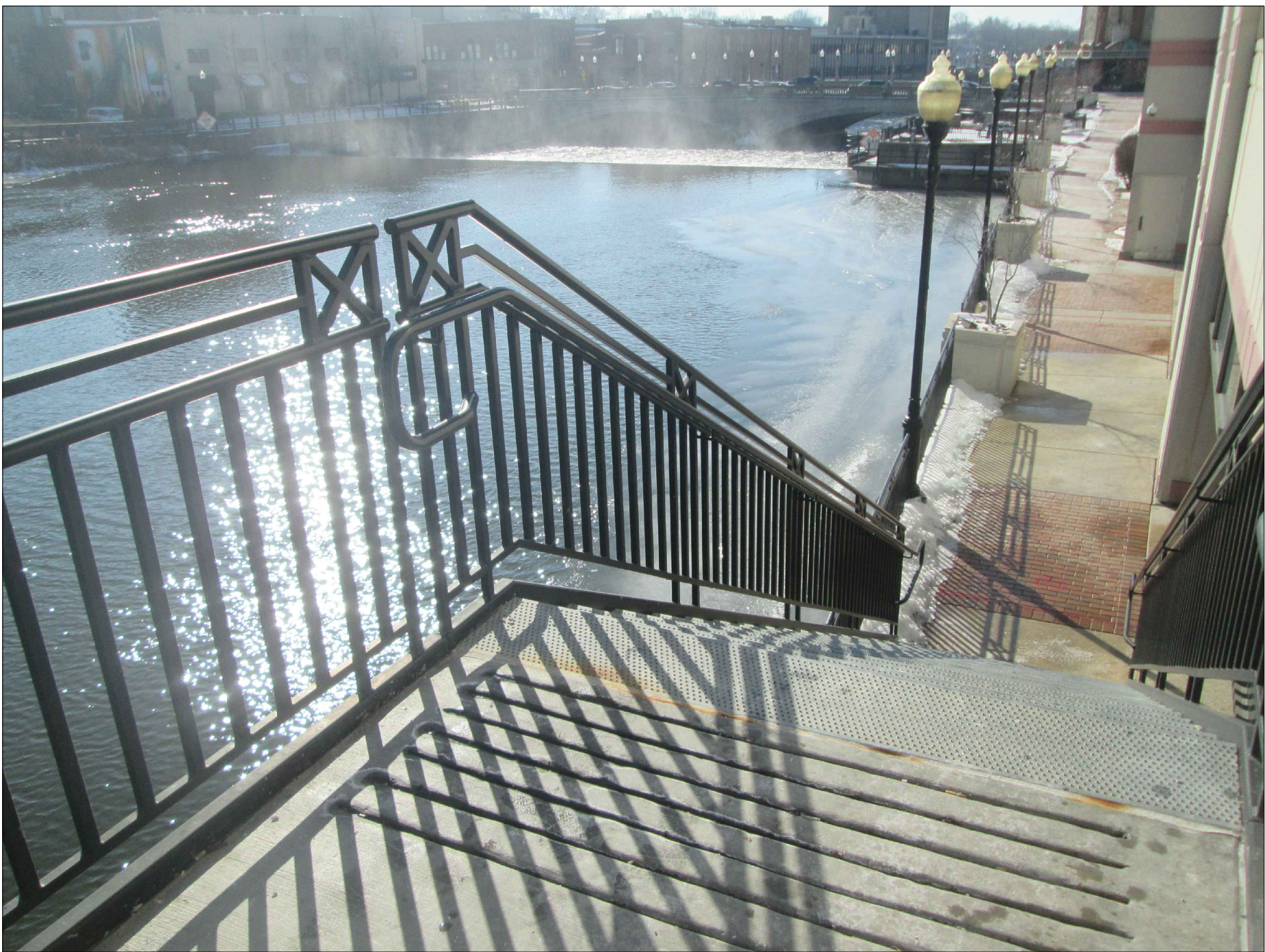
PHOTO 3 – EXISTING RAILING AT ADJACENT STAIRWAY
