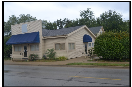
View looking northwest to the south and east elevations of the subject
