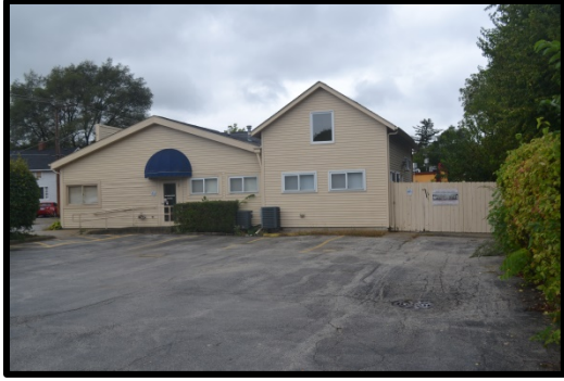
View of the east elevation of the subject
