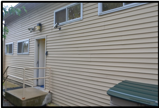
View of the north elevation of the subject
