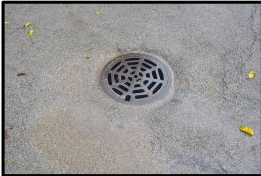
View of a storm sewer inlet in the parking lot
