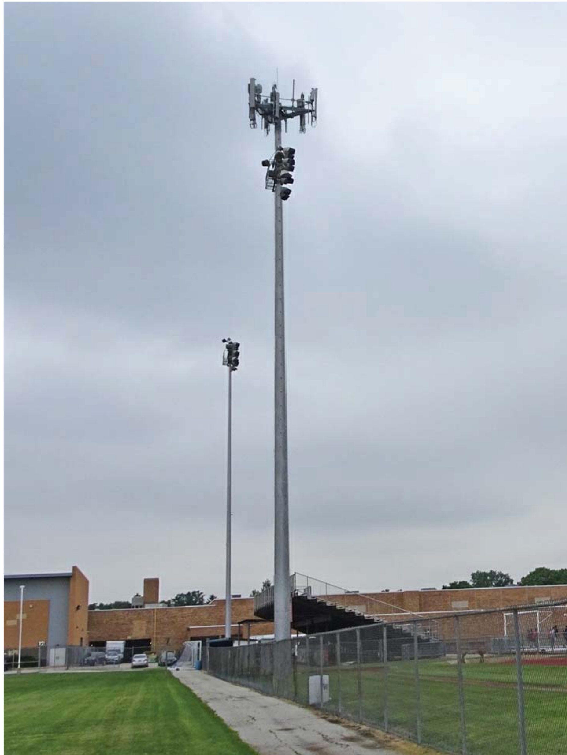
AURORA WEST HIGH SCHOOL LIGHT POLE CELL SITE
