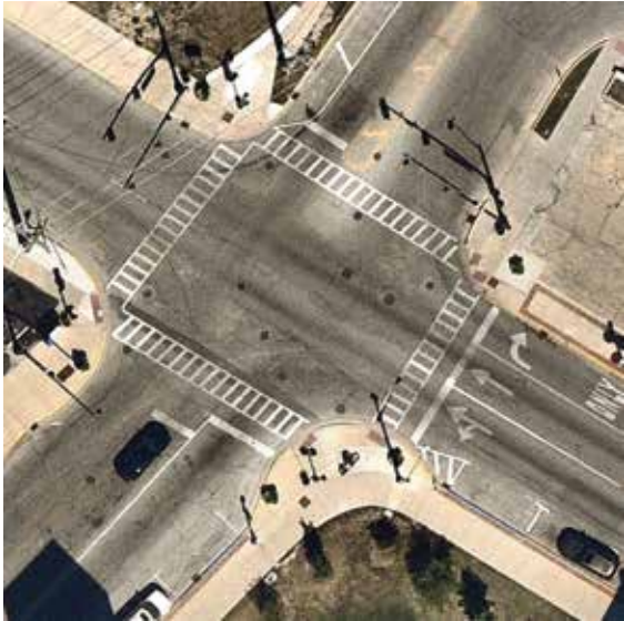
EXISTING INTERSECTION (W. NEW YORK/RIVER)
