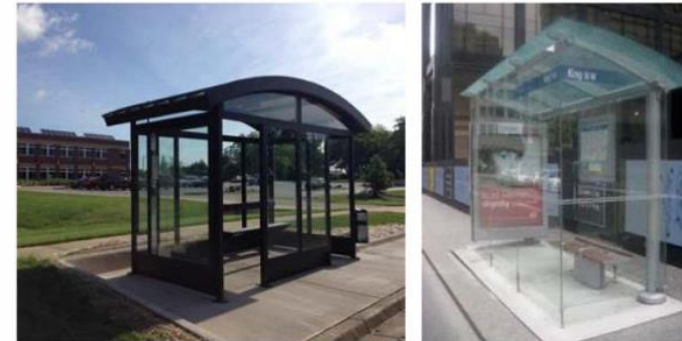
Examples of Bus Shelter
