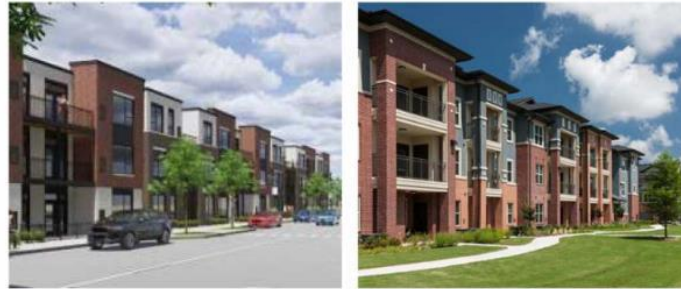
Examples of Residential buildings
