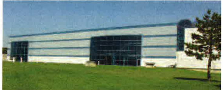
Aurora Water Treatment Facility
