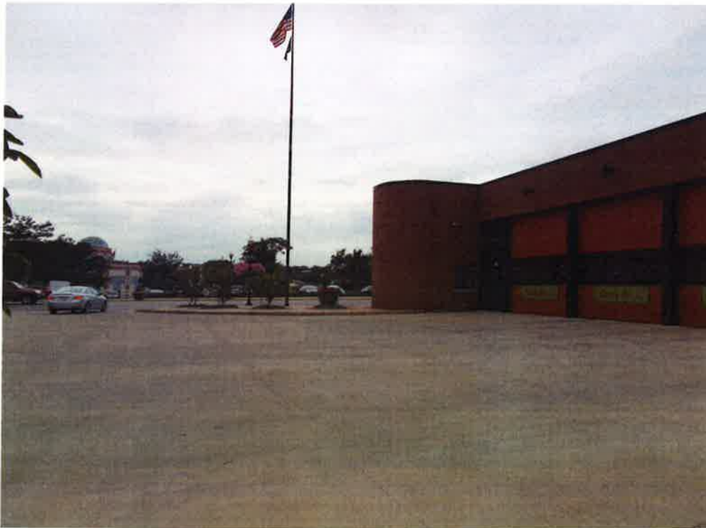
6. Central Fire Station west of the Subject Property.
