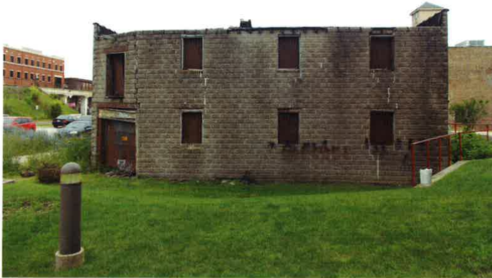
7. Looking south at the Subject Property.
