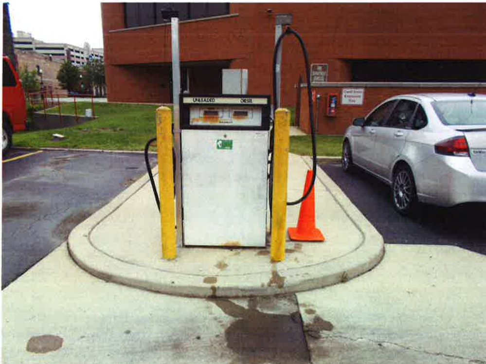
10. Gasoline and Diesel Fuel dispenser at the Central Fire Station.
