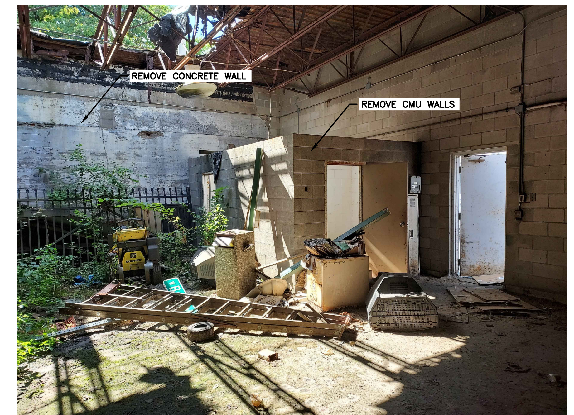
6 INTERIOR WALL NORTH & EAST
