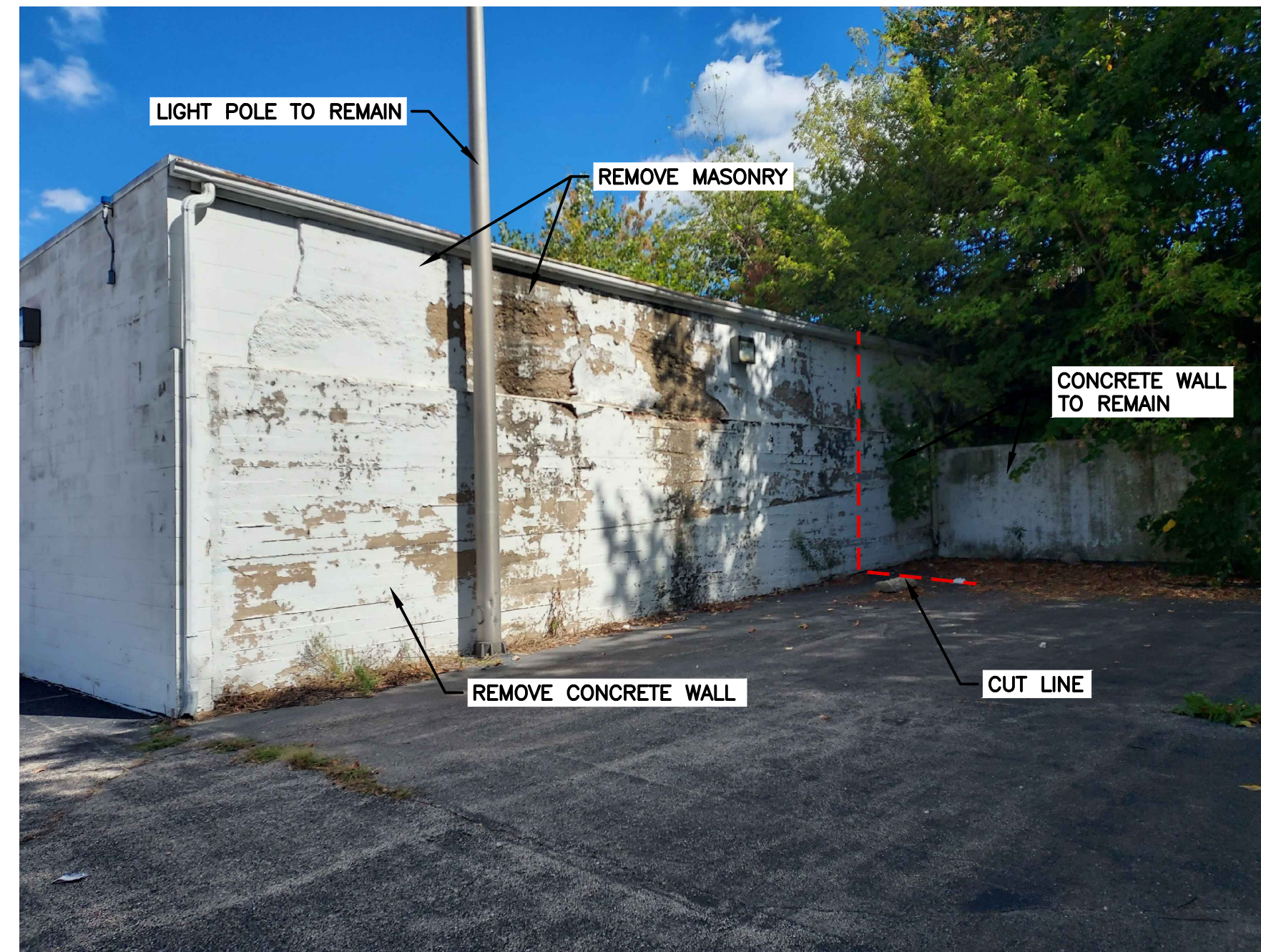
2 EXISTING MASONRY BUILDING WEST FACE
