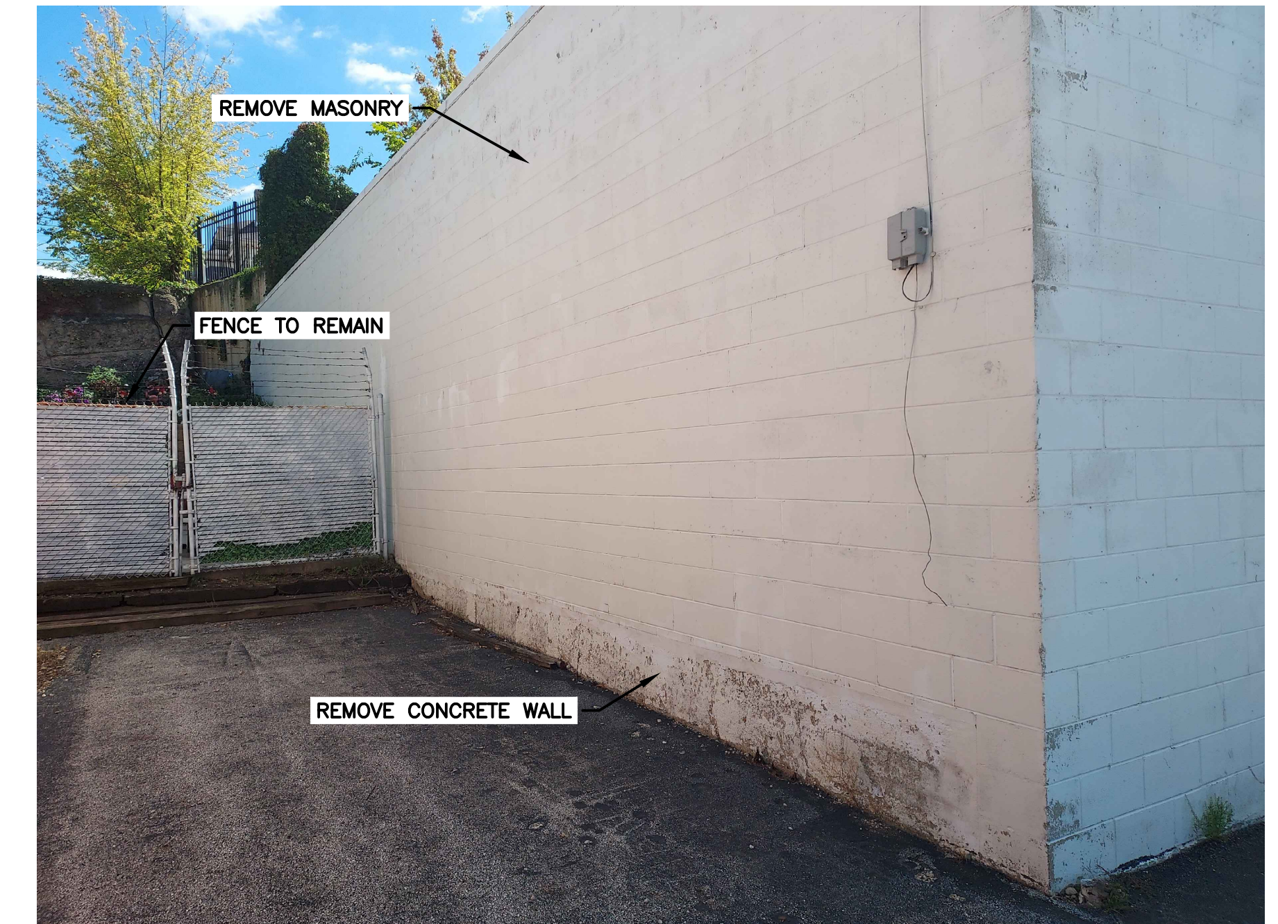
3 EXISTING MASONRY BUILDING EAST FACE
