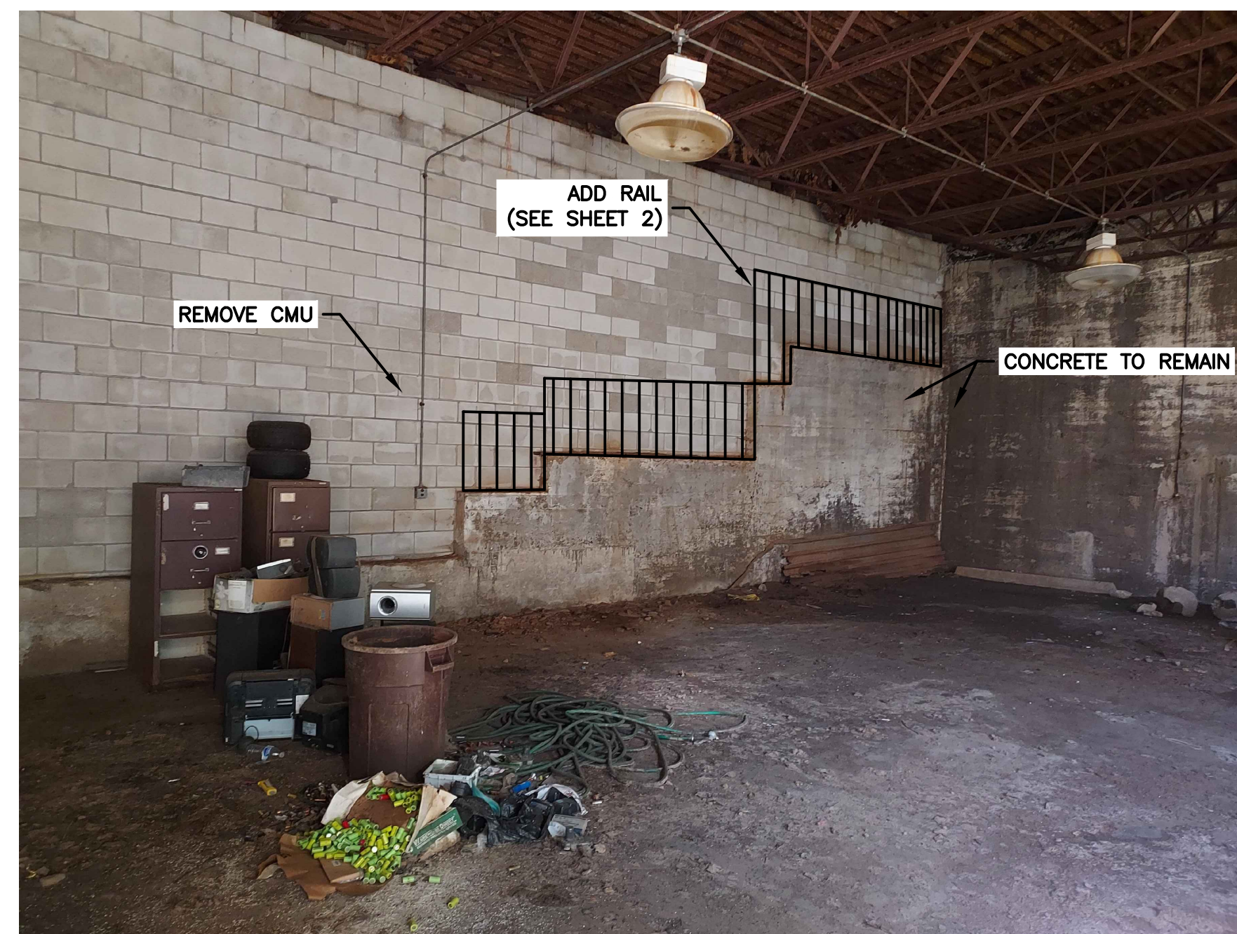
5 INTERIOR WALL - WEST
