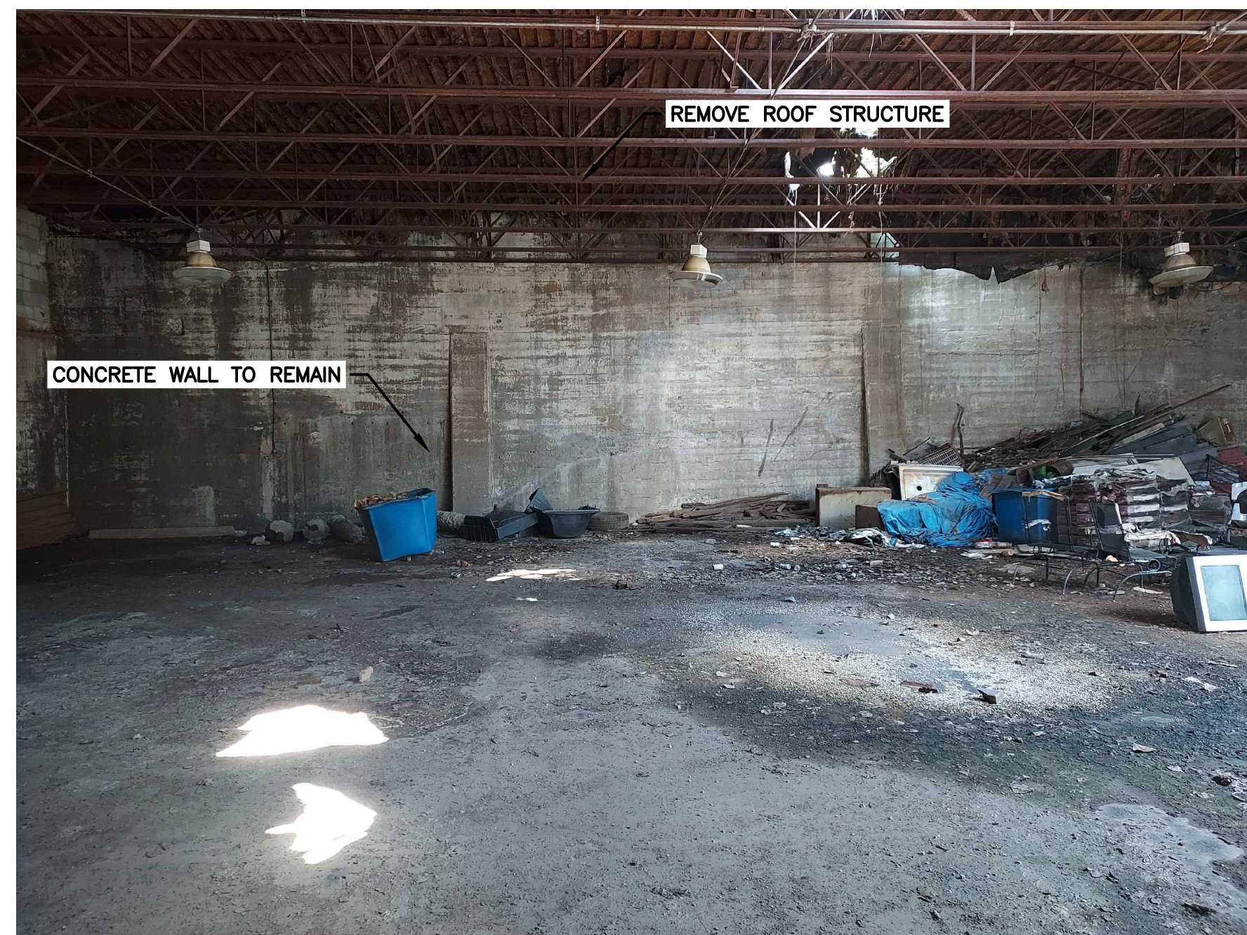
4 INTERNAL WALL - SOUTH
