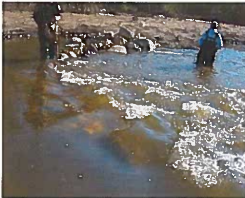
Riffle structure on the west branch of the DuPage River designed for canoe and kayak passage
