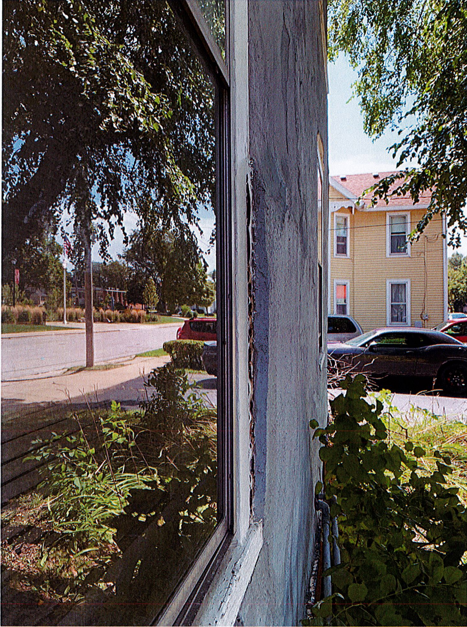
Same as above photo. West side of house.
