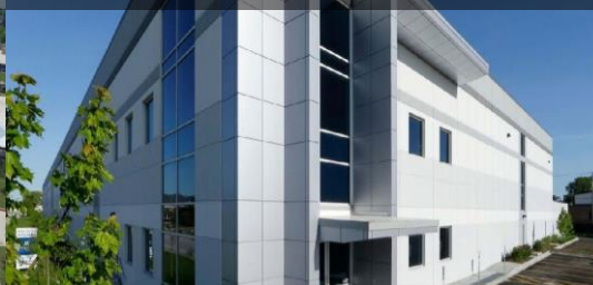
Stream Data Center Elk Grove Village, IL – 150,000 SF
