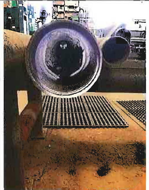
Heavy encrustation on ID of column (typ.)
