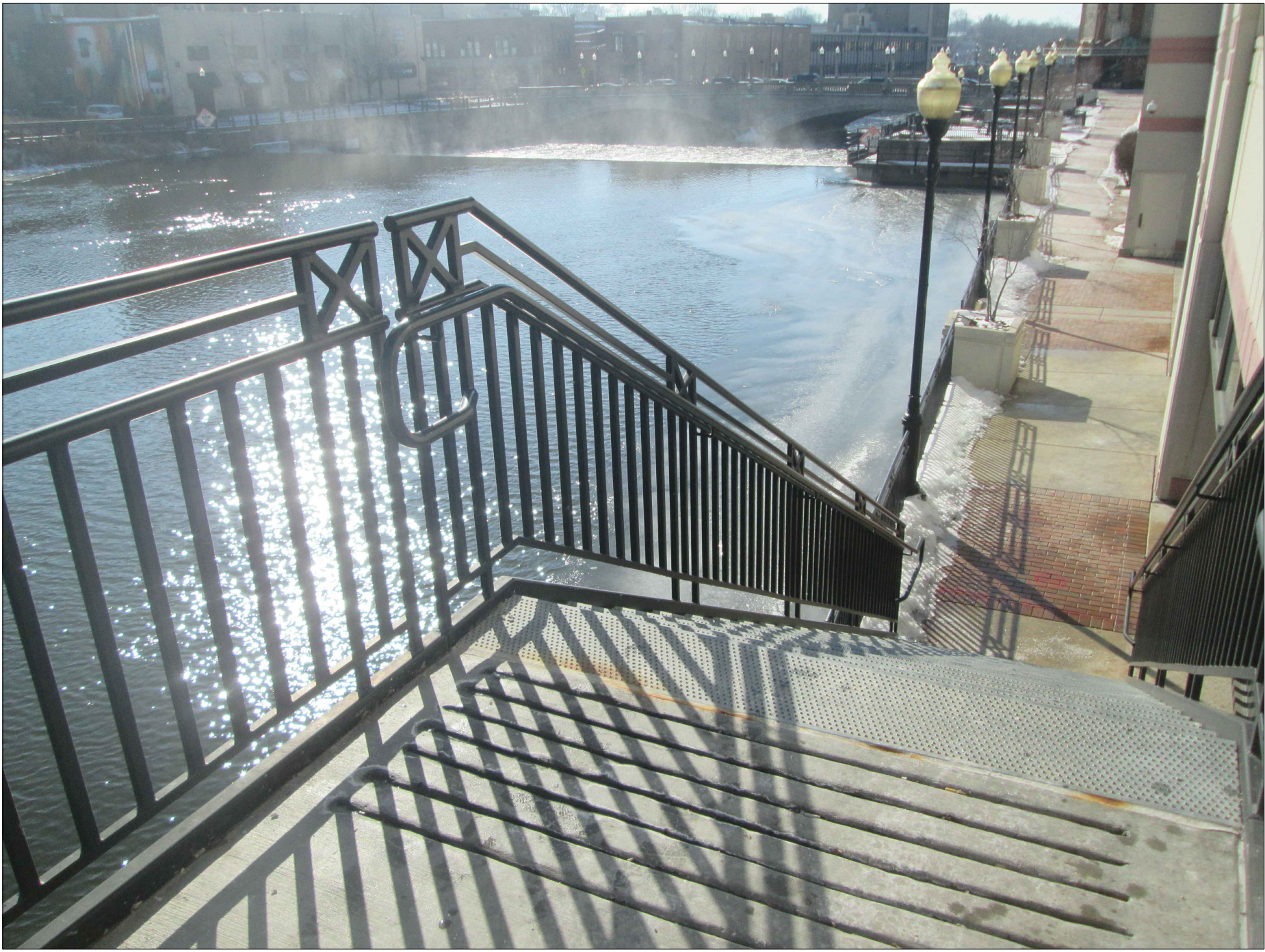
PHOTO 3 – EXISTING RAILING AT ADJACENT STAIRWAY
